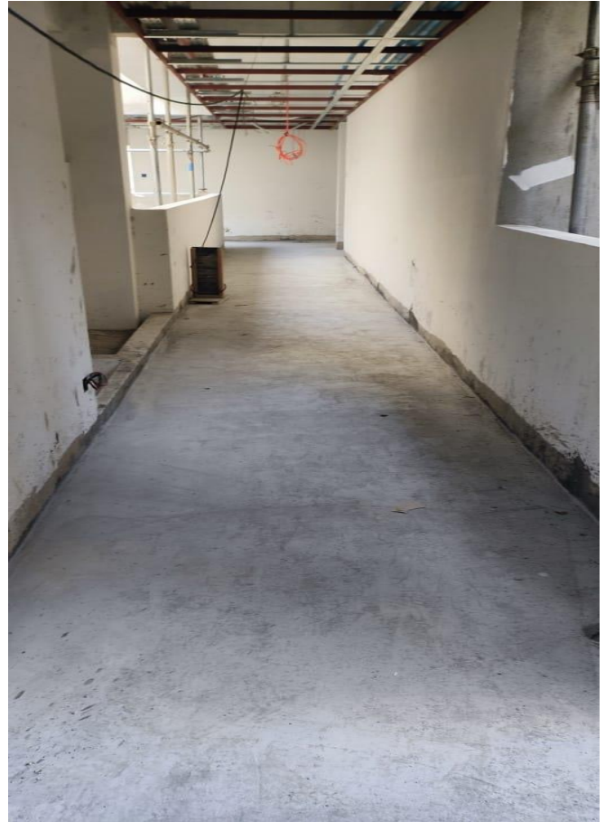
Common area screeding and ceiling work
