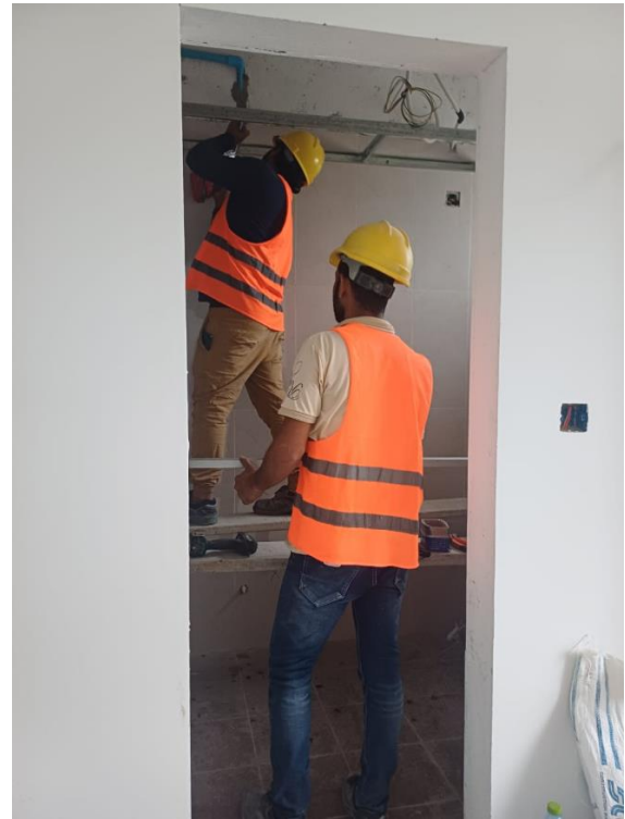
Apartment plumbing work
