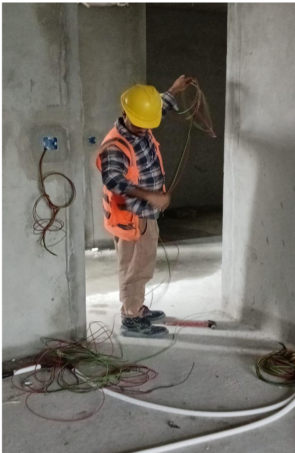
12 th floor wiring work
