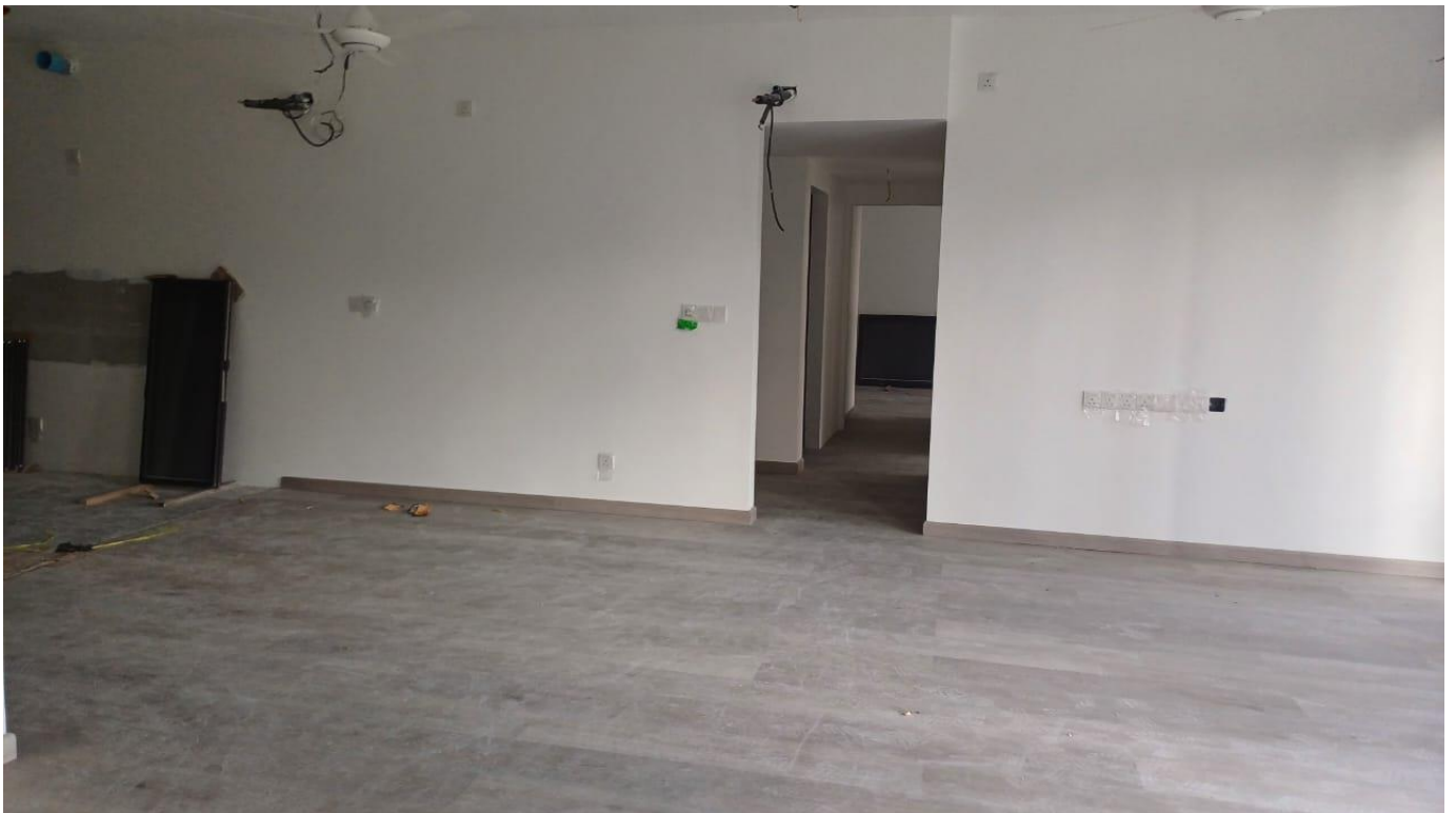
10th floor painting,ceiling,SPC and kitchen tile work
