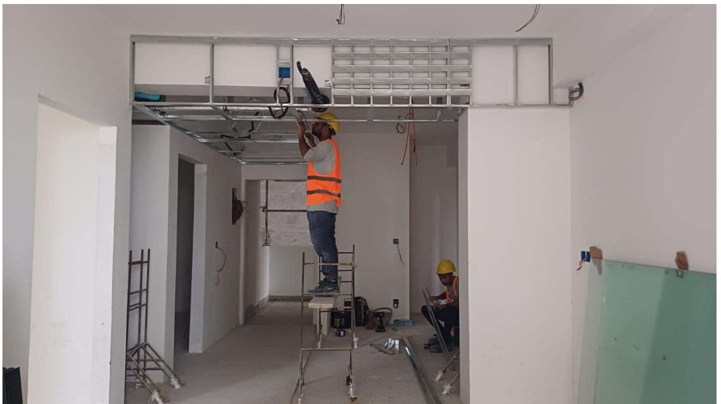
Apartment ceiling work
