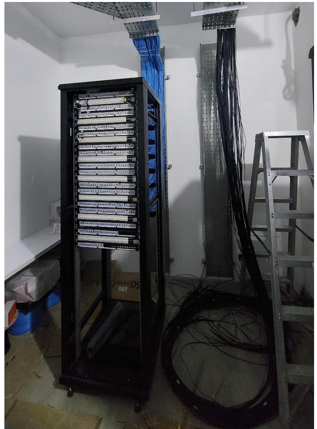
Data and telephone cable laying
