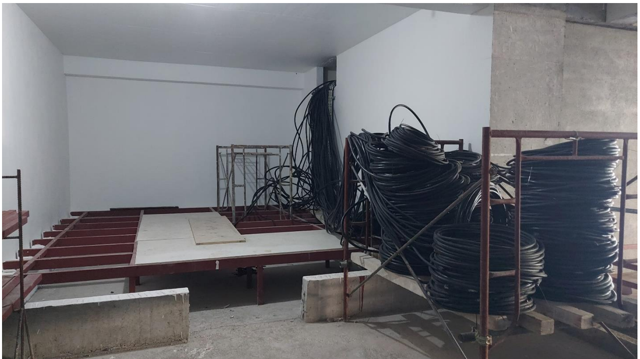
Electrical Main cable laying
