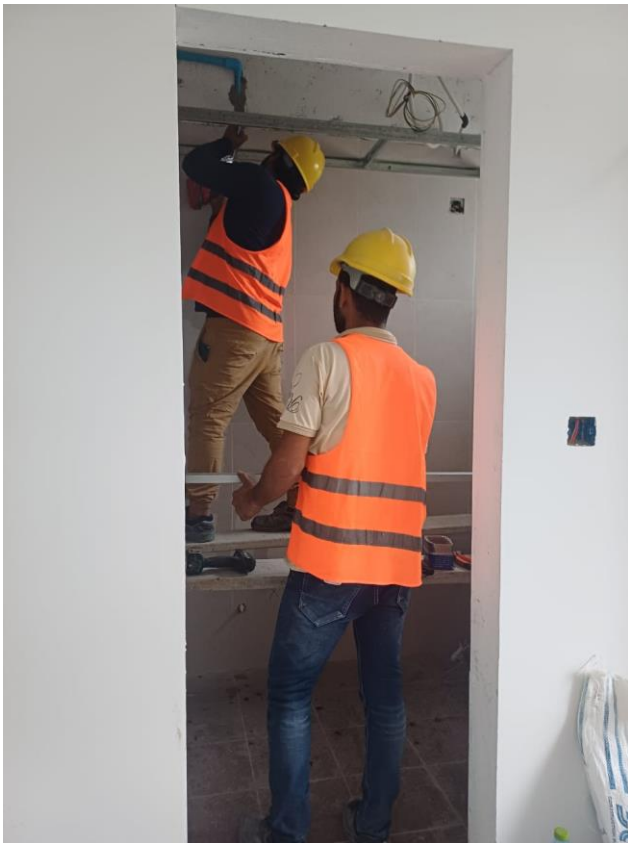
Toilet false ceiling work
