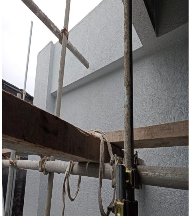
External primer and painting work
