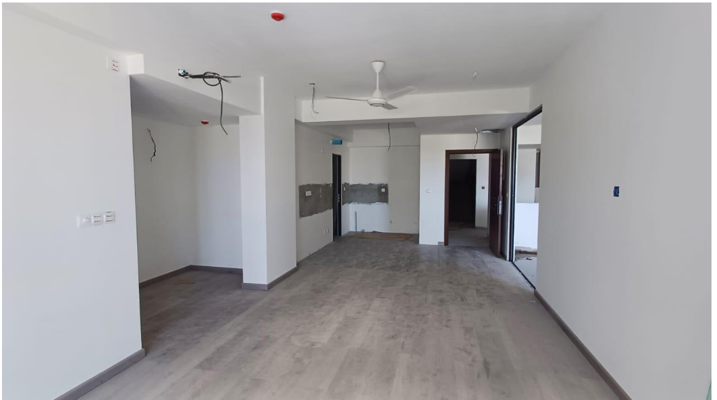
4 th floor SPC and WPC door fixing
