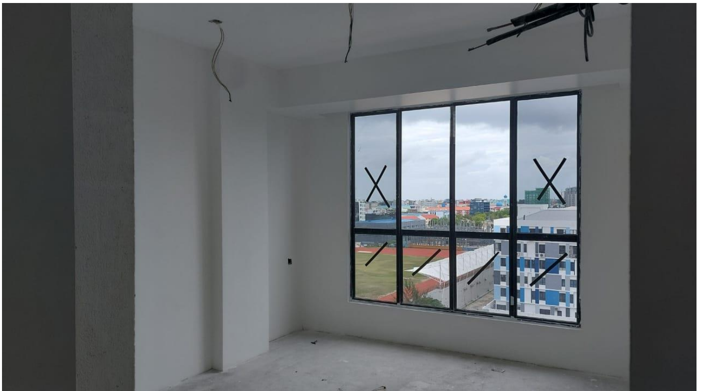
11 th floor Aluminium Windows fixing
