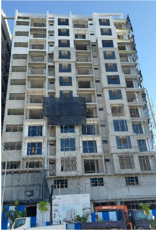
WPC, Windows and sliding door fixing
