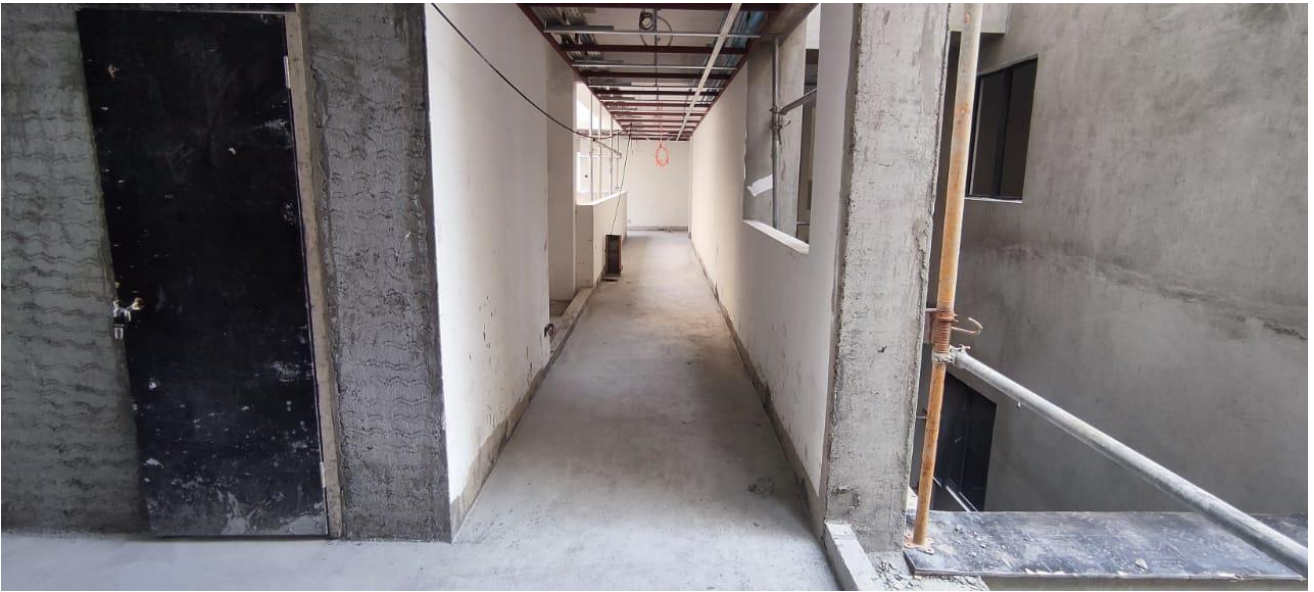
Common area screeding
