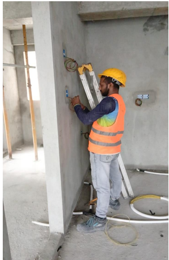
Apartment wiring work
