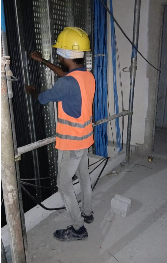
2 nd to 12 th floor main cable laying
