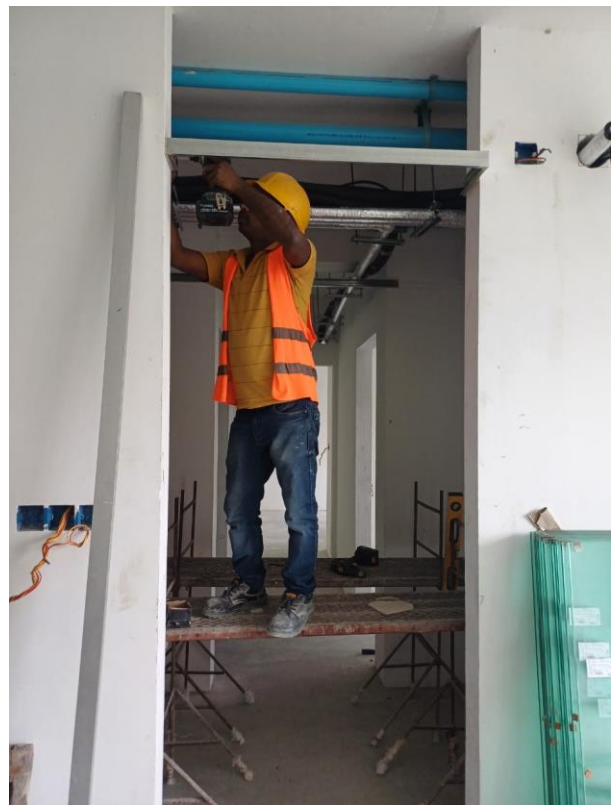
Apartment false ceiling work
