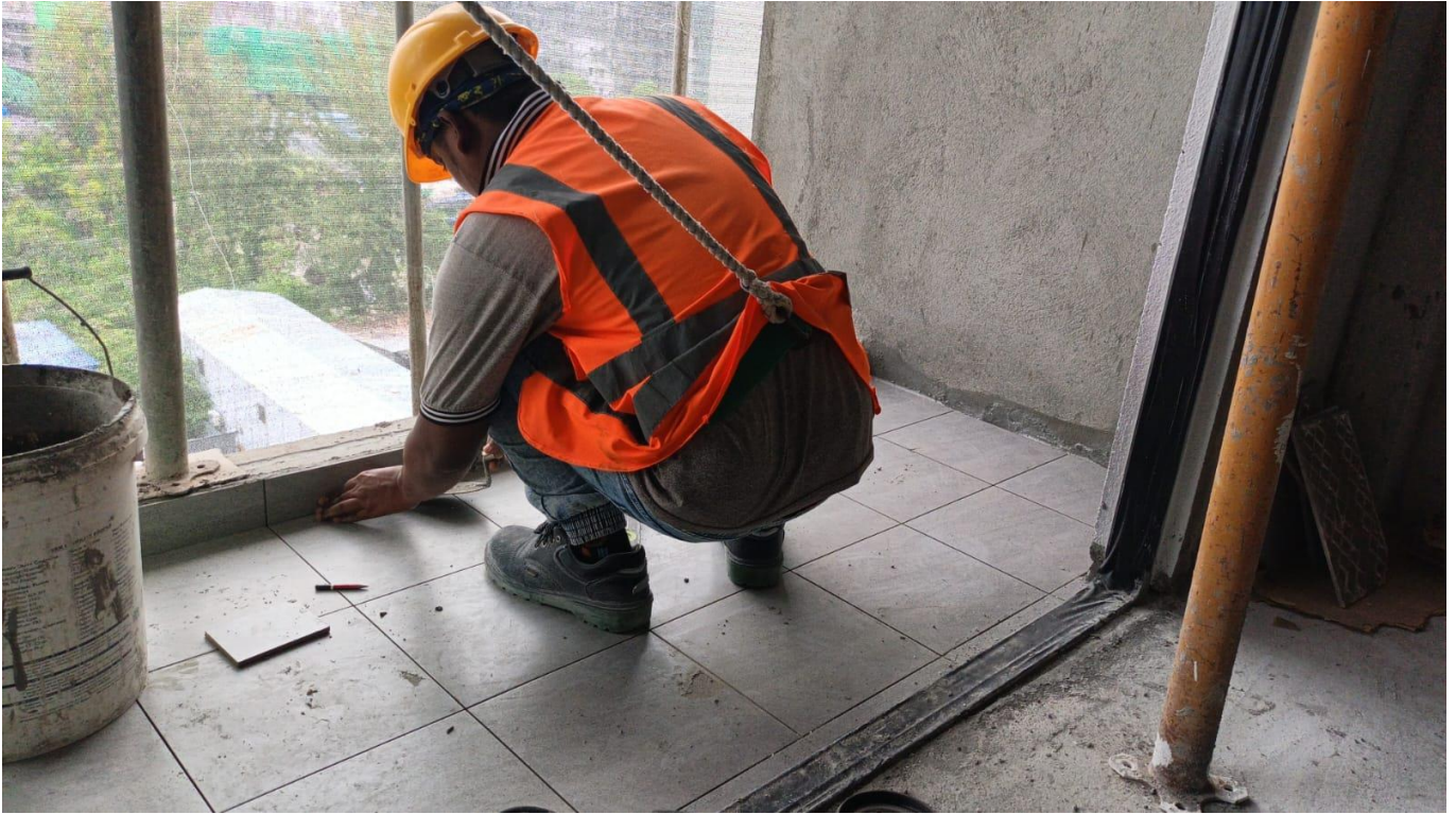
Balcony tile laying
