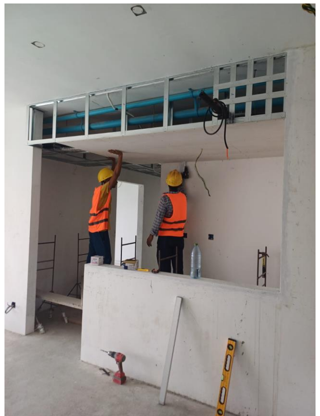
Apartment false ceiling work
