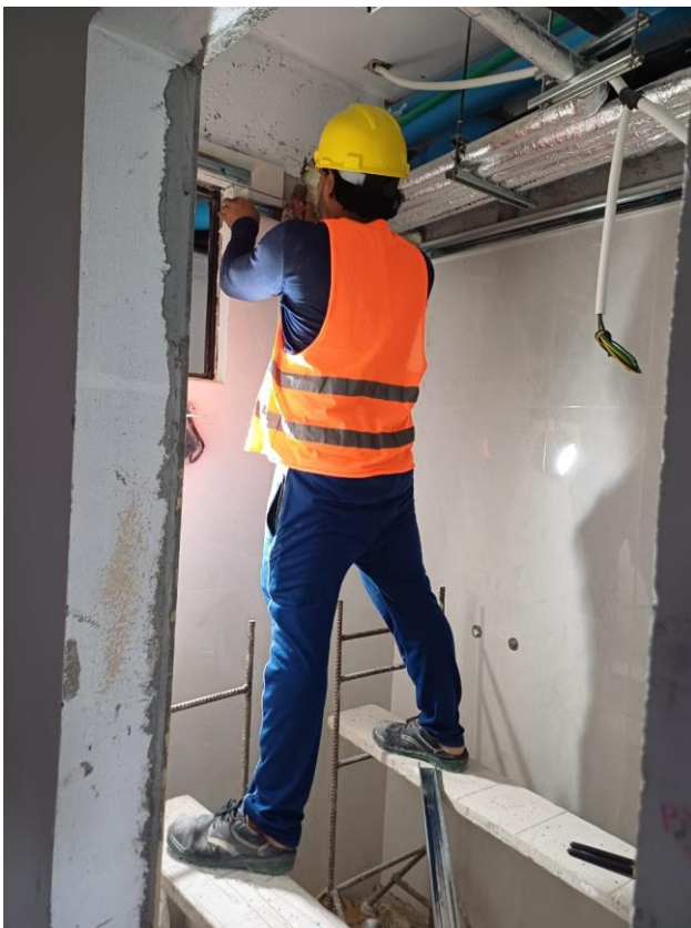
Toilet tile work fixing
