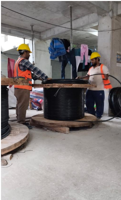
Electrical Main cable laying
