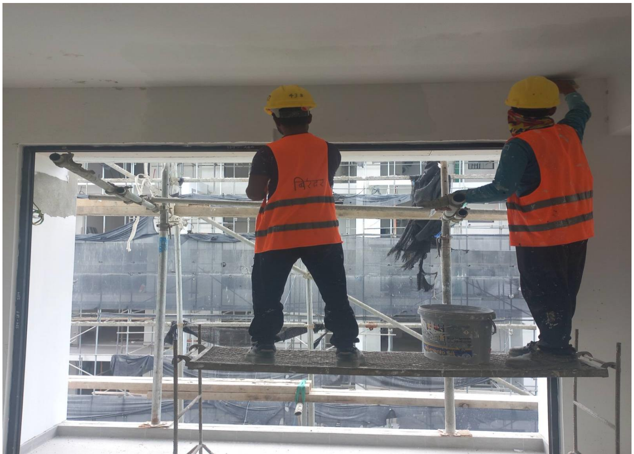
AC ledge masonry and waterproofing
