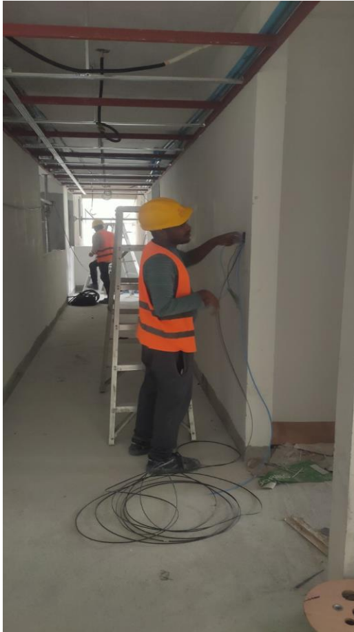
Common area ceiling wiring work
