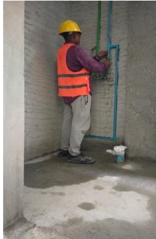
12 th floor plumbing work
