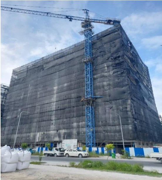
Safety Net installation
