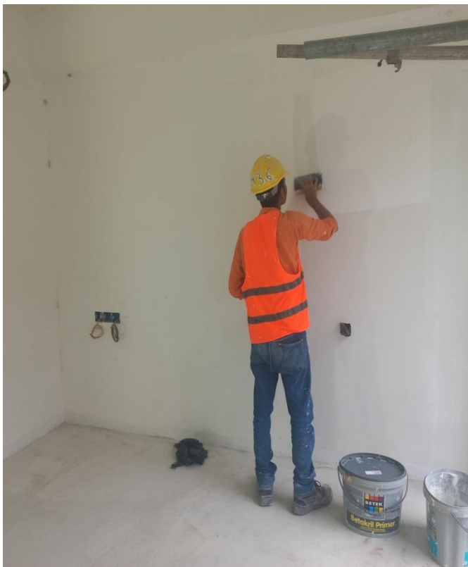
4 th floor Apartment internal putty & painting
