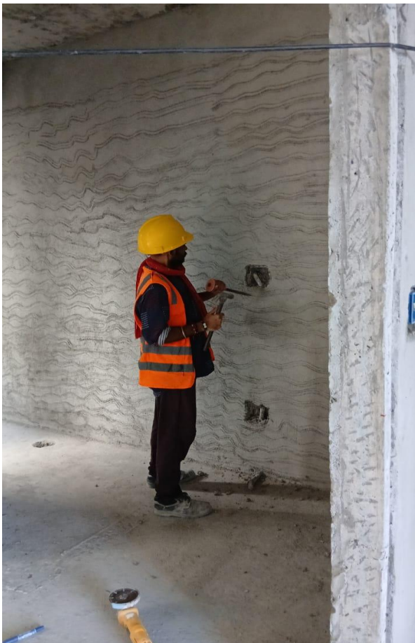
12 th floor socket fixing
