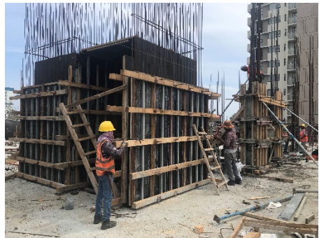
4th Floor Lift Wall Formworks
