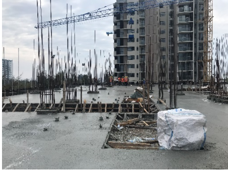
5th Floor Slab Concrete Casting
