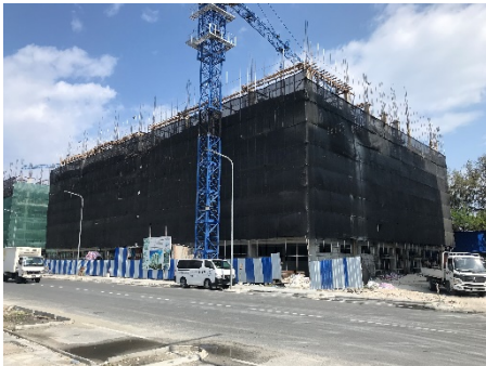
Safety Net Installation
