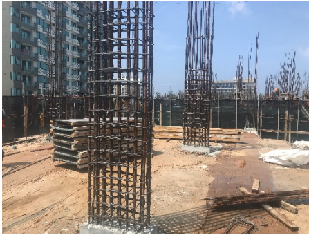
4th Columns Reinforcement
