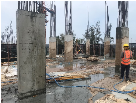
4th Floor Column Concrete Casting
