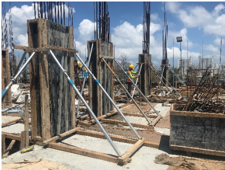
5th Floor Column Formworks
