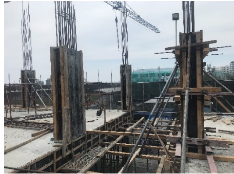
4th Columns Formworks
