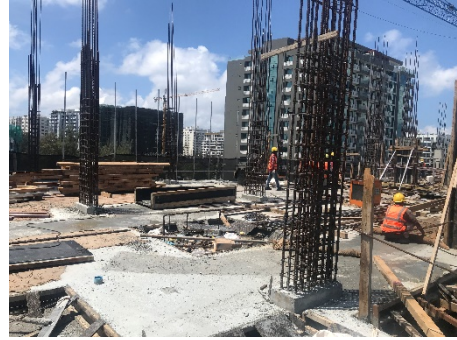
5th Floor Column Reinforcement
