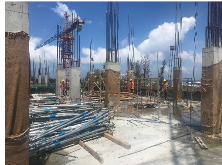
5th Floor Column Concrete Casting
