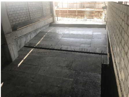
Basement Ramp Formworks
