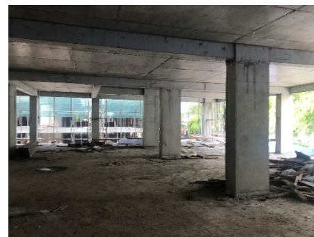
First Floor Slab De-shuttering
