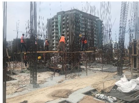
3rd Floor Column & Lift Reinforcement
