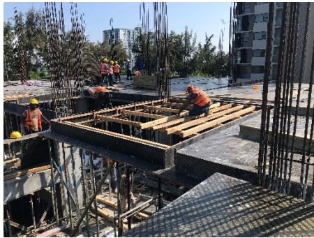
3rd Floor Slab and Beam Formworks
