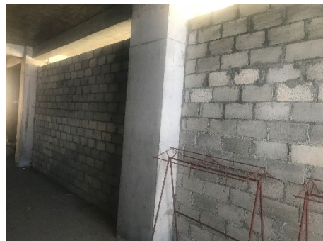
Ground Floor Slab Masonry Work
