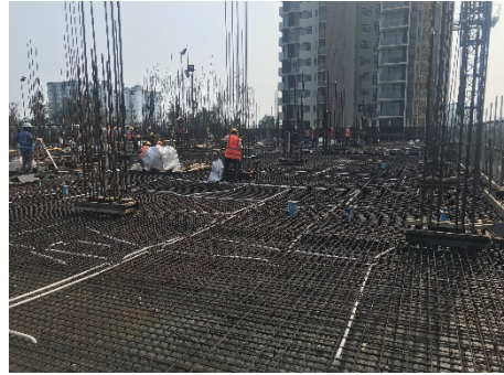
4th Floor Slab and Beam Reinforcement
