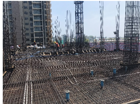
3rd Floor Slab and Beam Reinforcement
