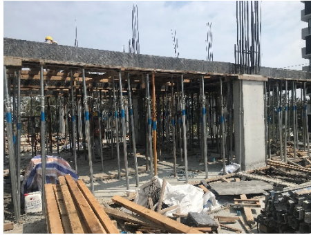
4th Floor Slab and Beam Formworks
