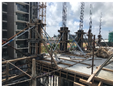
3rd Floor Column Formworks
