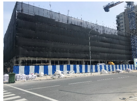
Safety Net Installation
