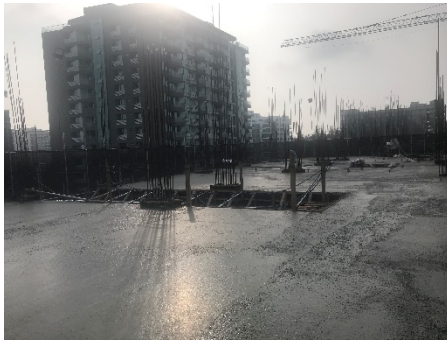
4th Floor Slab Concrete Casting
