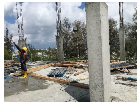
3rd Floor Column Concrete Casting
