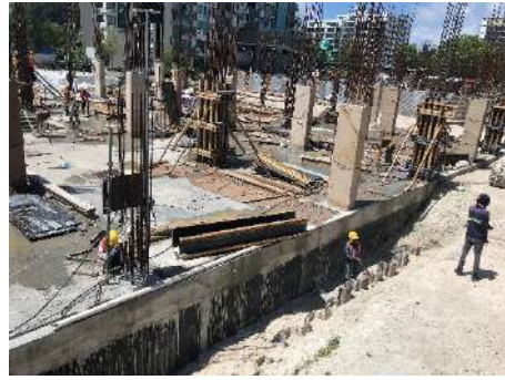
Ground Column Concrete Casting
