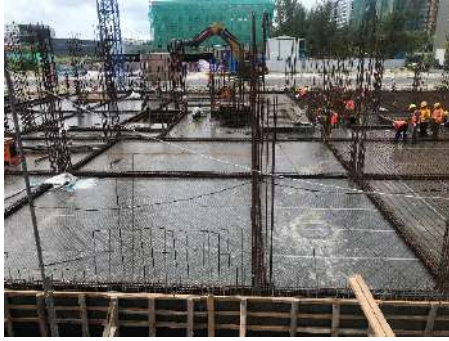
Ground Slab and Beam Formworks
