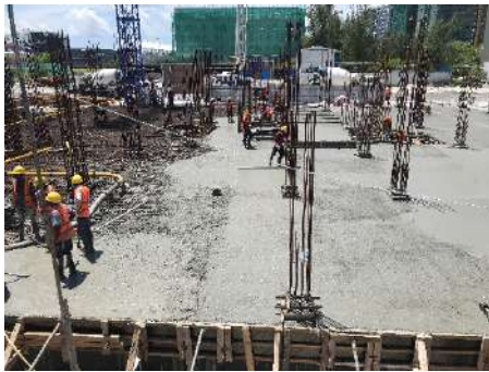
Ground Slab Concrete Casting
