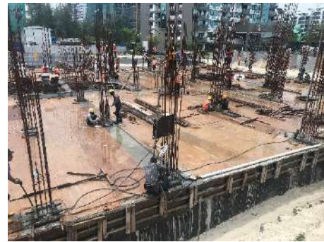
Ground Column Reinforcement
