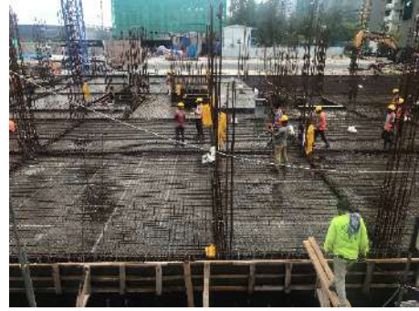
Ground Slab and Beam Reinforcement
