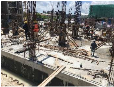
Ground Column Formworks
