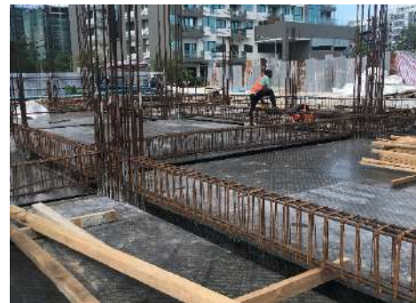
Beams (Ground) Reinforcement
