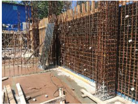
Retaining Wall Reinforcement
