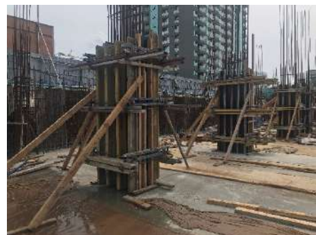
Columns (Below Grd) Formworks
