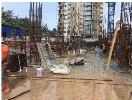
Columns (Below Grd) Reinforcement
