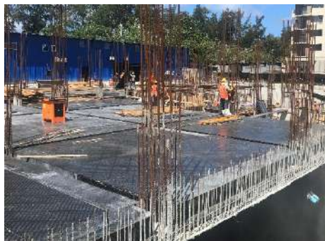
Slab & Beams (Ground) Formworks
