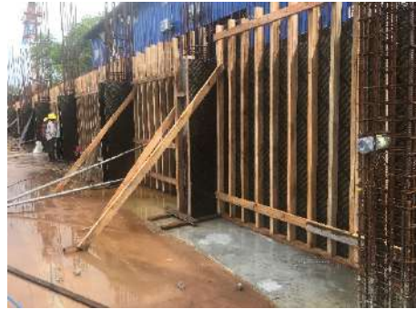
Retaining Wall Formworks
