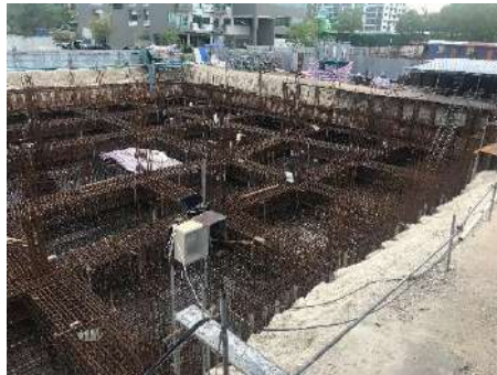
Foundation Beam Reinforcement
