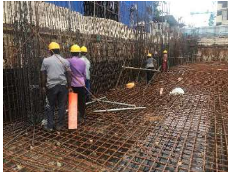
Retaining Wall Reinforcement
