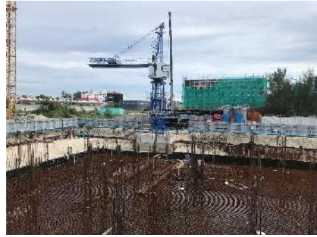
Tower Crane Erection
