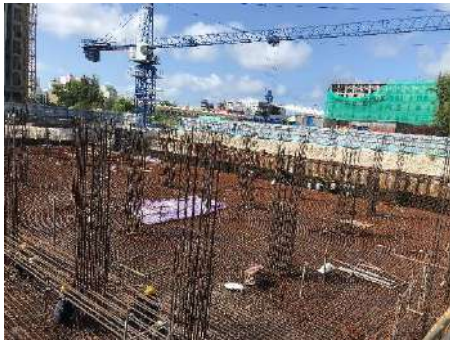
Columns Reinforcement
