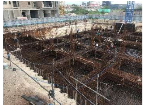
Foundation Beam Reinforcement
