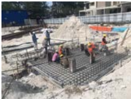
Tower Crane Foundation
