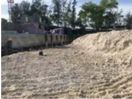
Excavation Works (1 meter Level)
