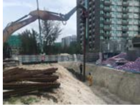
Sheet Pile Driving
