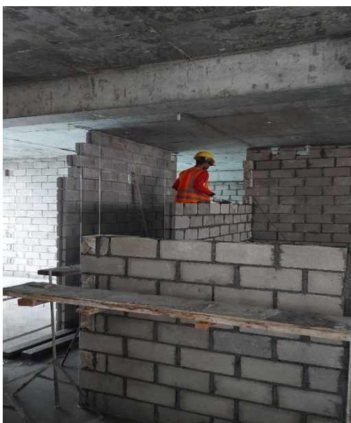
12 th floor block work
