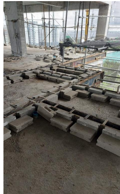
11 th floor kicker concrete
