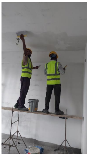
3 rd floor putty work continuous
