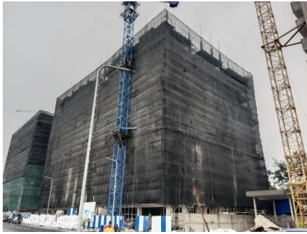
Safety Net installation
