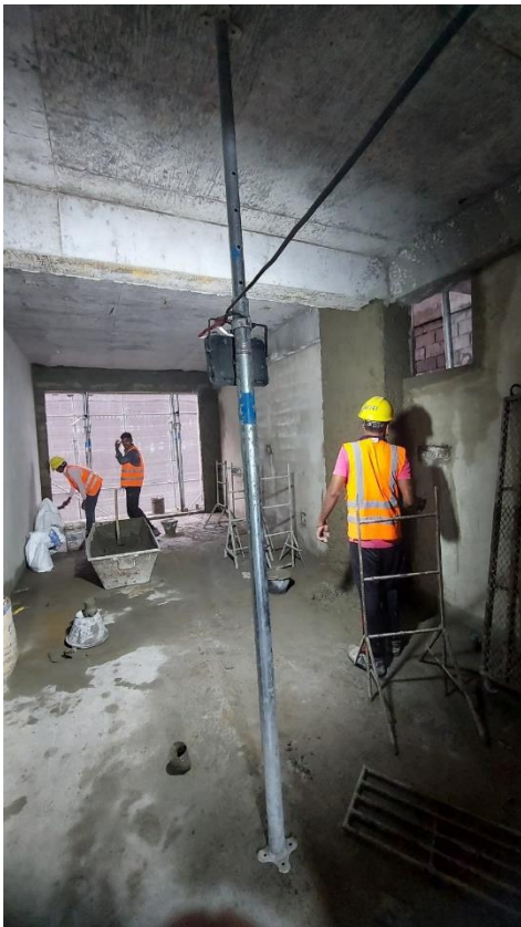
10 th floor plastering work continuous
