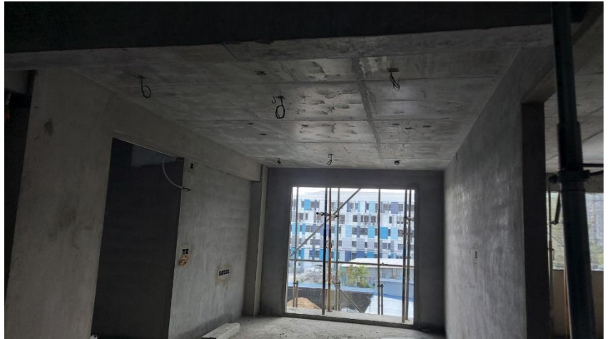
3 rd floor wiring work completed
