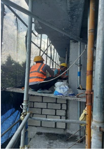
Front view elevation block work
