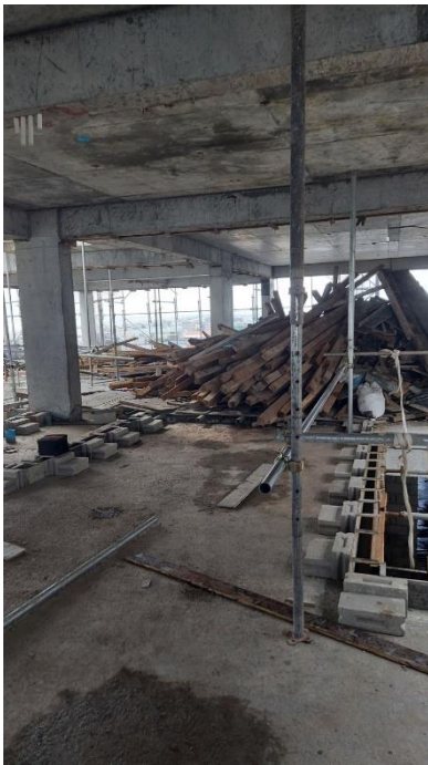
12 th floor kicker concrete
