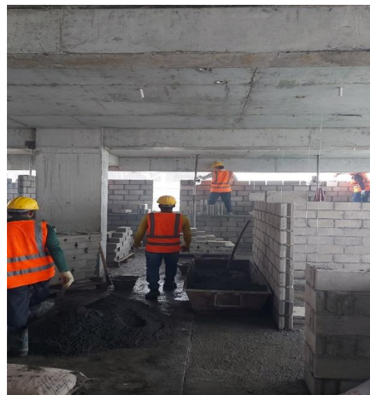
12 th floor block work
