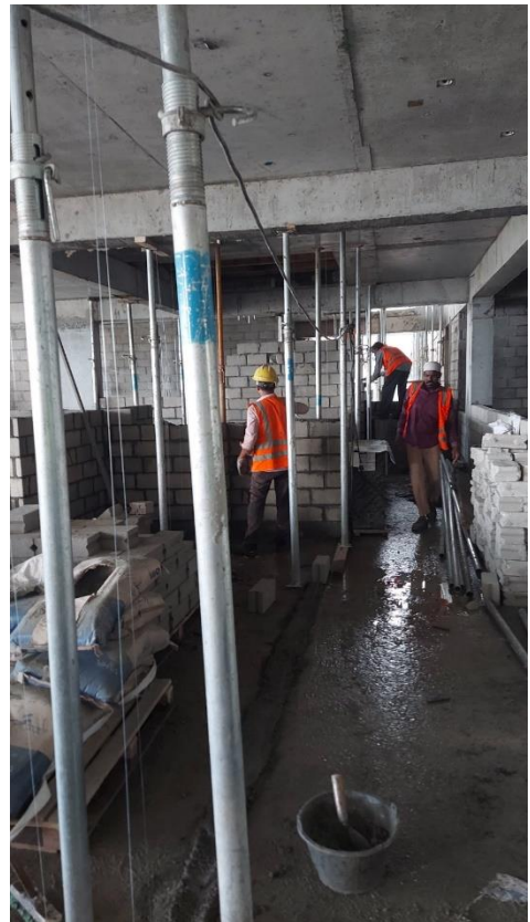
11 th floor block work continuous
