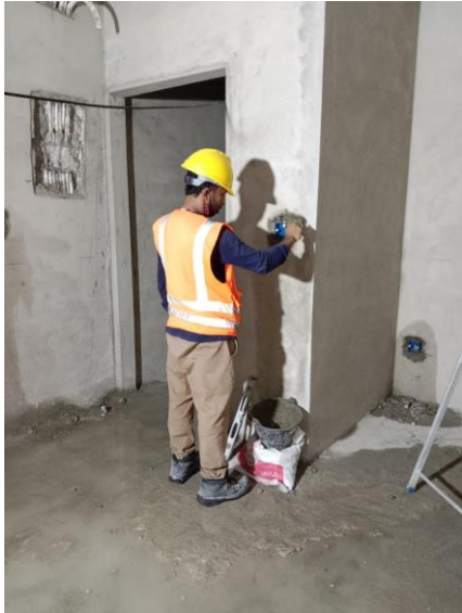
6 th floor socket box fixing
