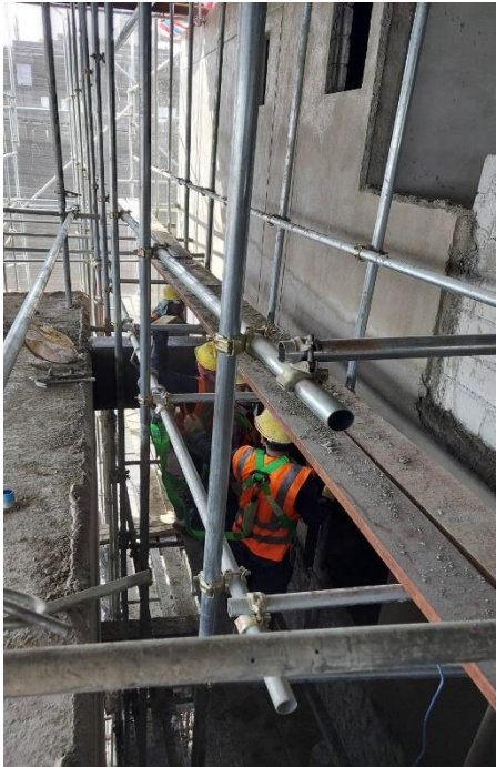
Elevation E5,E6 external plastering
