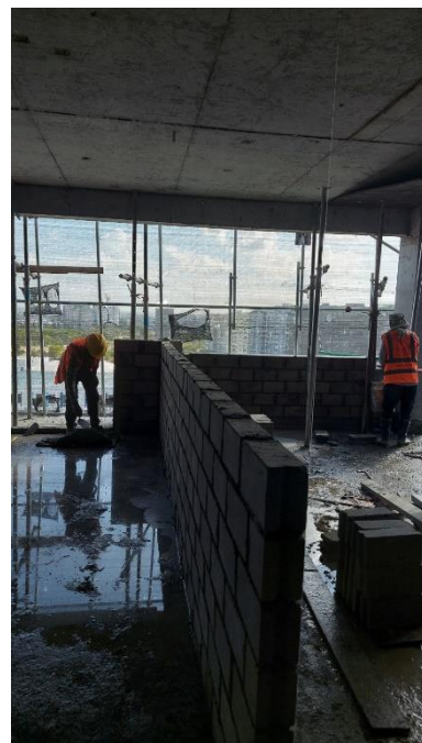
12 th floor block work continue
