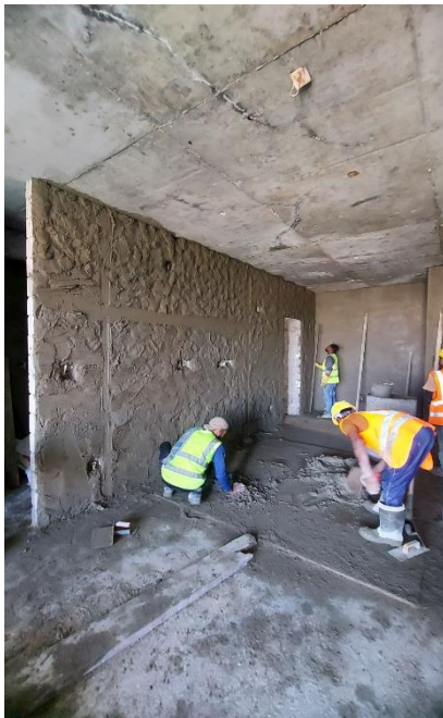
12 th floor plastering work continuous
