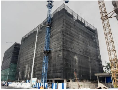
Safety Net installation
