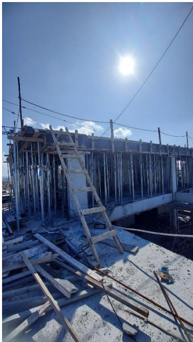
Mumty slab RCC concrete
