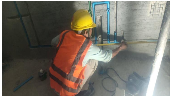
2 nd floor plumbing work completed
