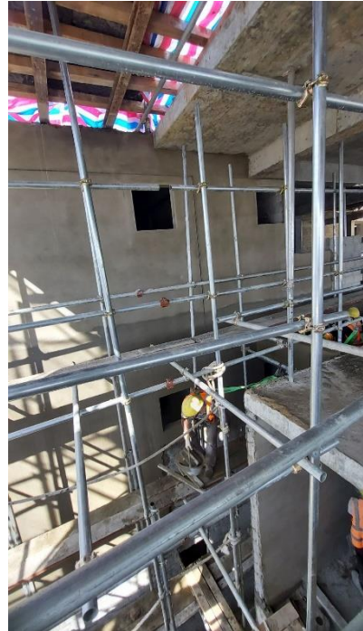
Elevation E7,E8 external plastering
