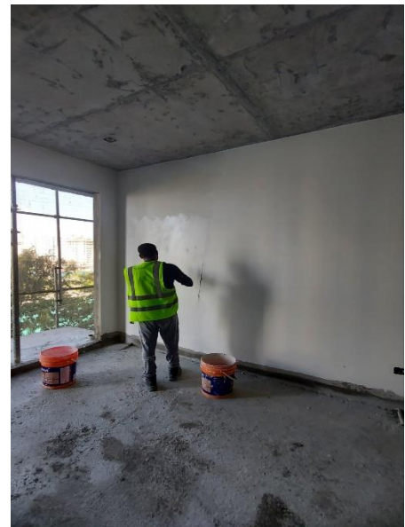
4 th floor putty work
