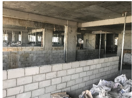
5th Floor Blocks Laying
