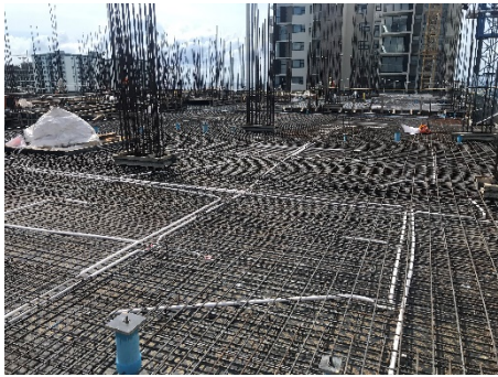
9th Floor Beam & Slab Reinf.
