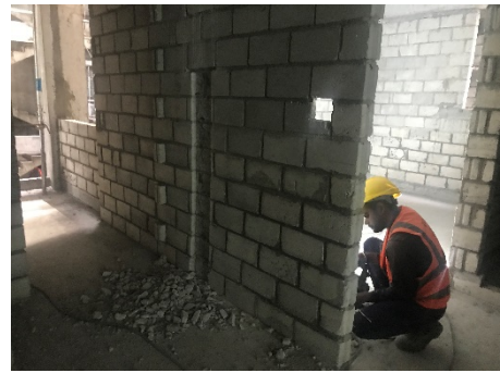
3rd Floor Electrical Wall Chasing
