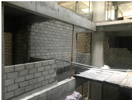
4th Floor Blocks Laying
