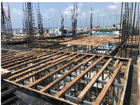
10th Floor Beam & Slab Formworks
