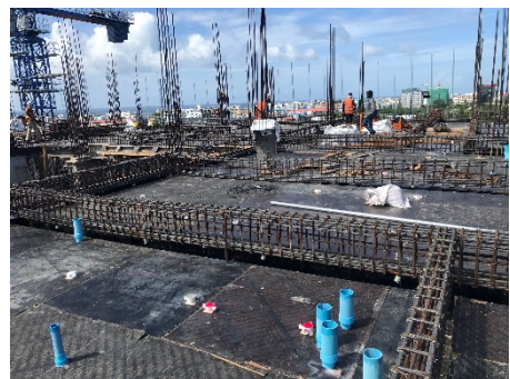
10th Floor Beam Reinforcement
