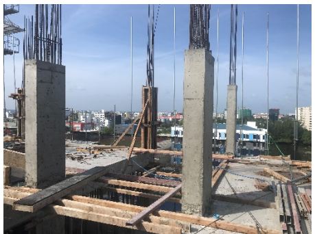
9th Floor Column Concrete
