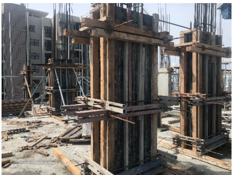
9th Floor Column Formworks
