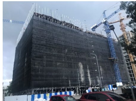
Safety Net Installation
