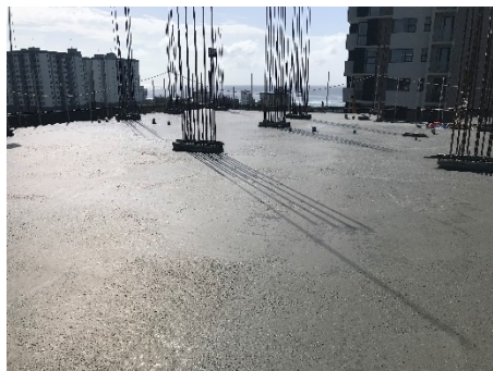
9th Floor Slab Concrete Casting
