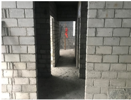
2nd Floor Block Laying
