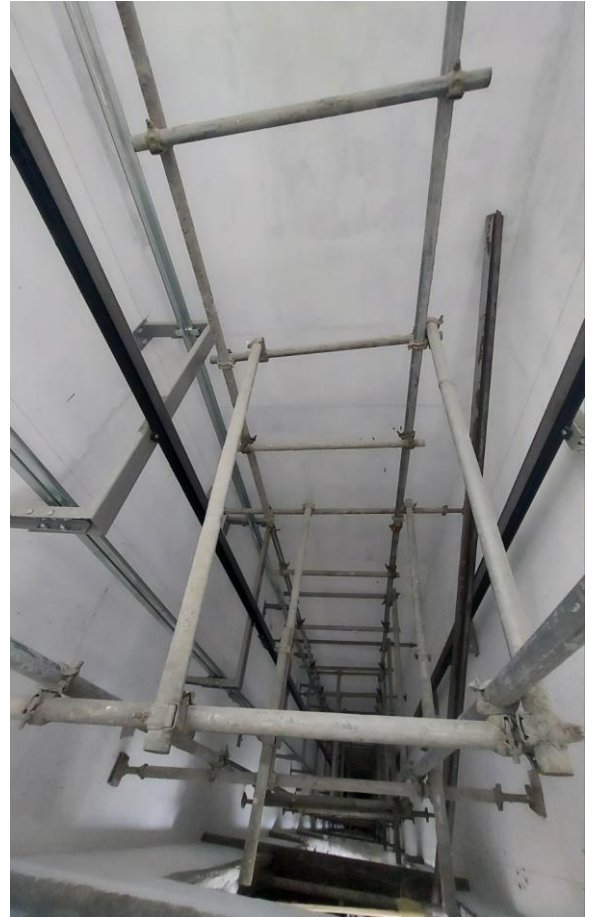
Lift frame work
