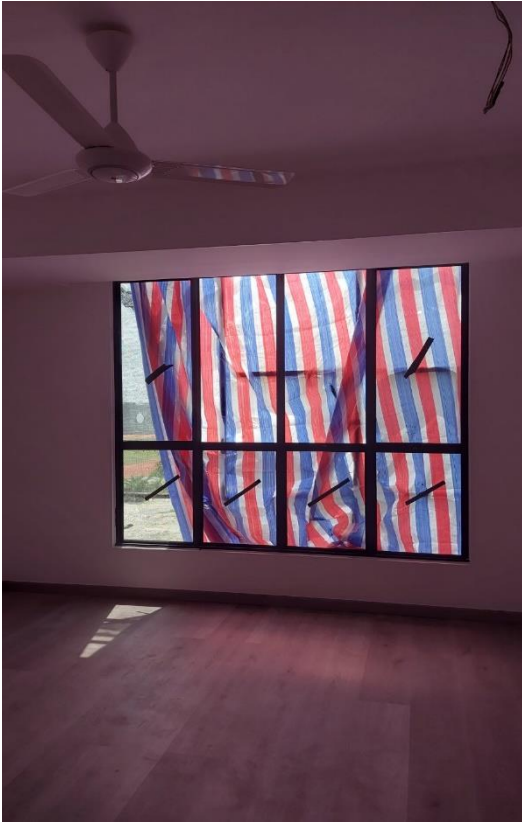
12 th floor windows fixing
