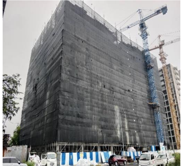
Safety Net Installation
