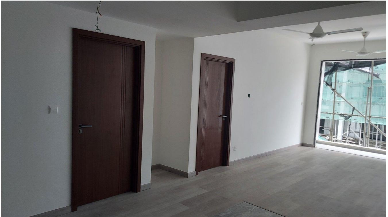
3 rd floor apartment door fixing
