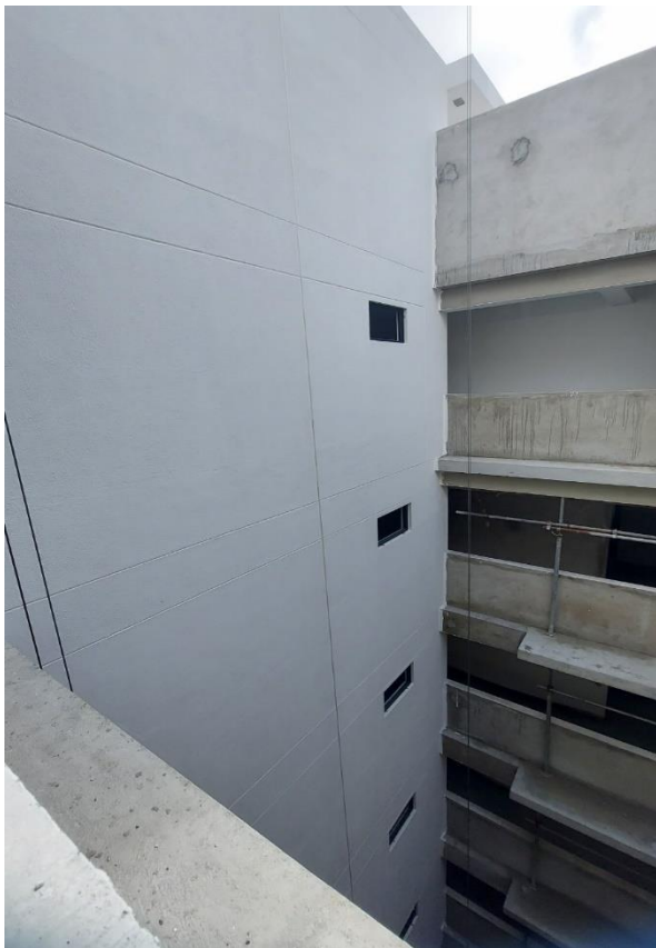
Big air well area external texture painting
