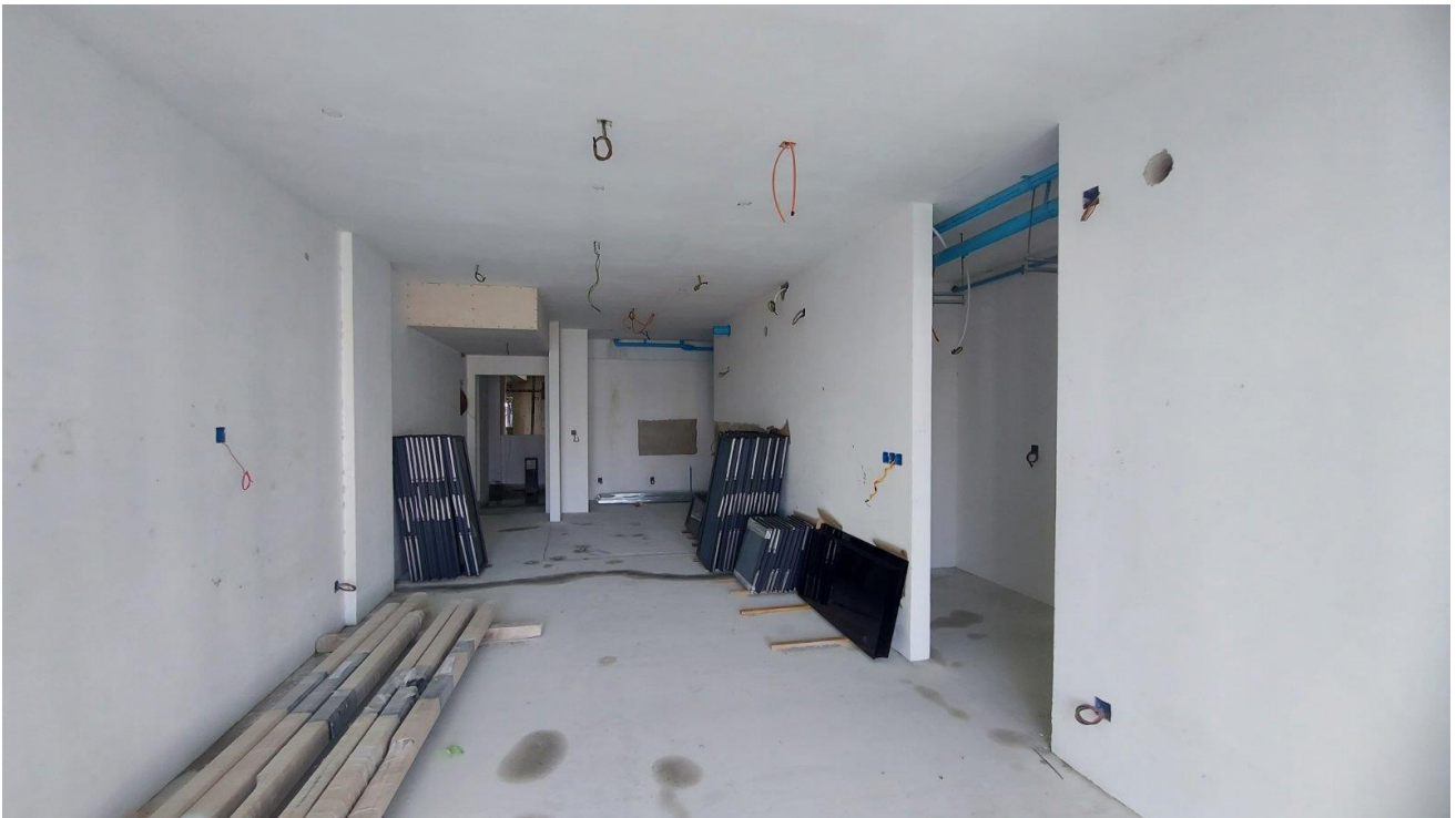
12 th floor Putty work
