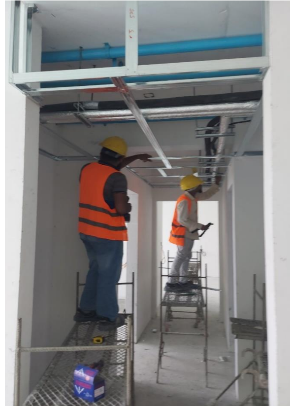
12 th floor apartment ceiling frame work
