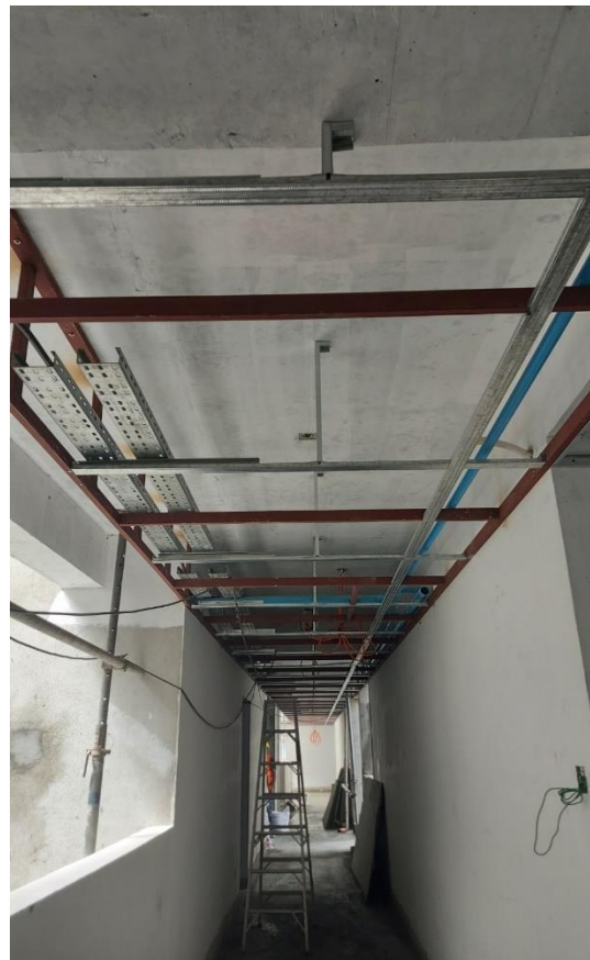
11 th floor common area cable tray fixing
