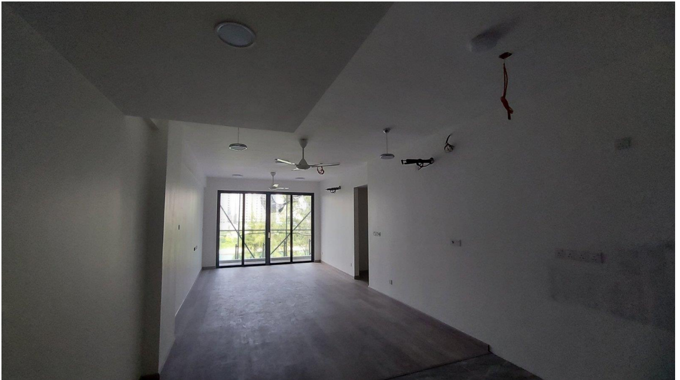
3 rd floor fan, ceiling, putty light and emulsion work
