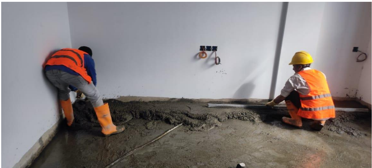
11 th floor common area and apartment screeding work
