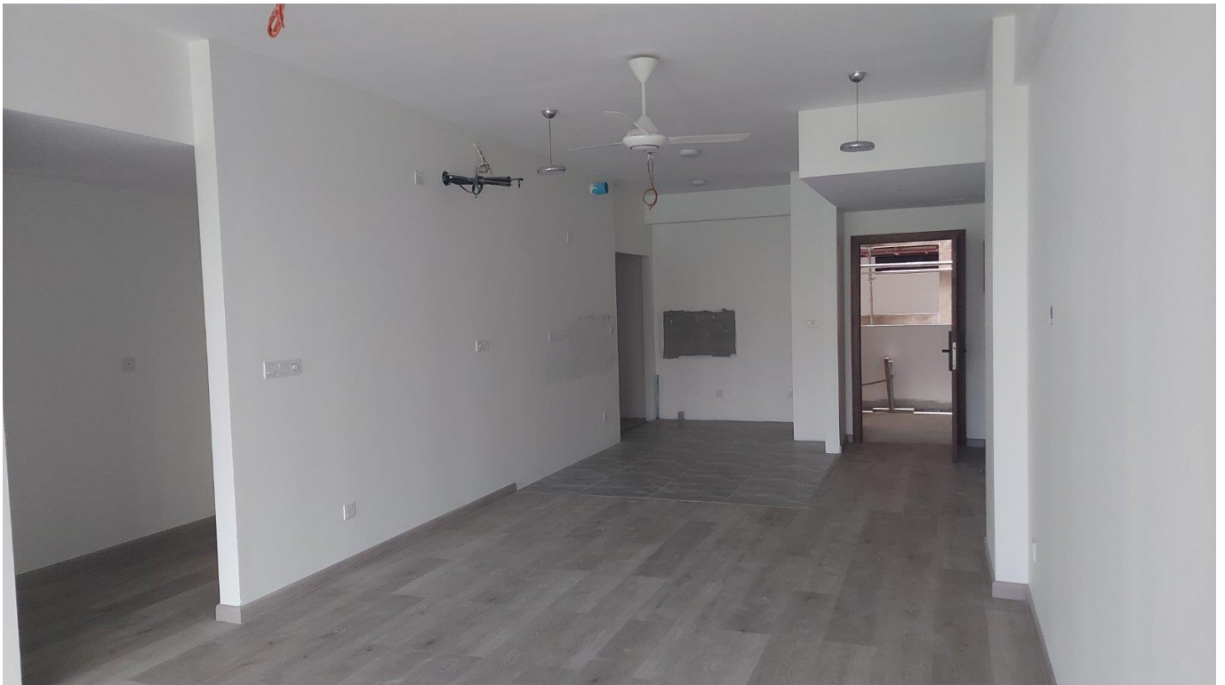
3 rd floor SPC and Tile work
