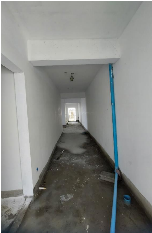
Penthouse putty work
