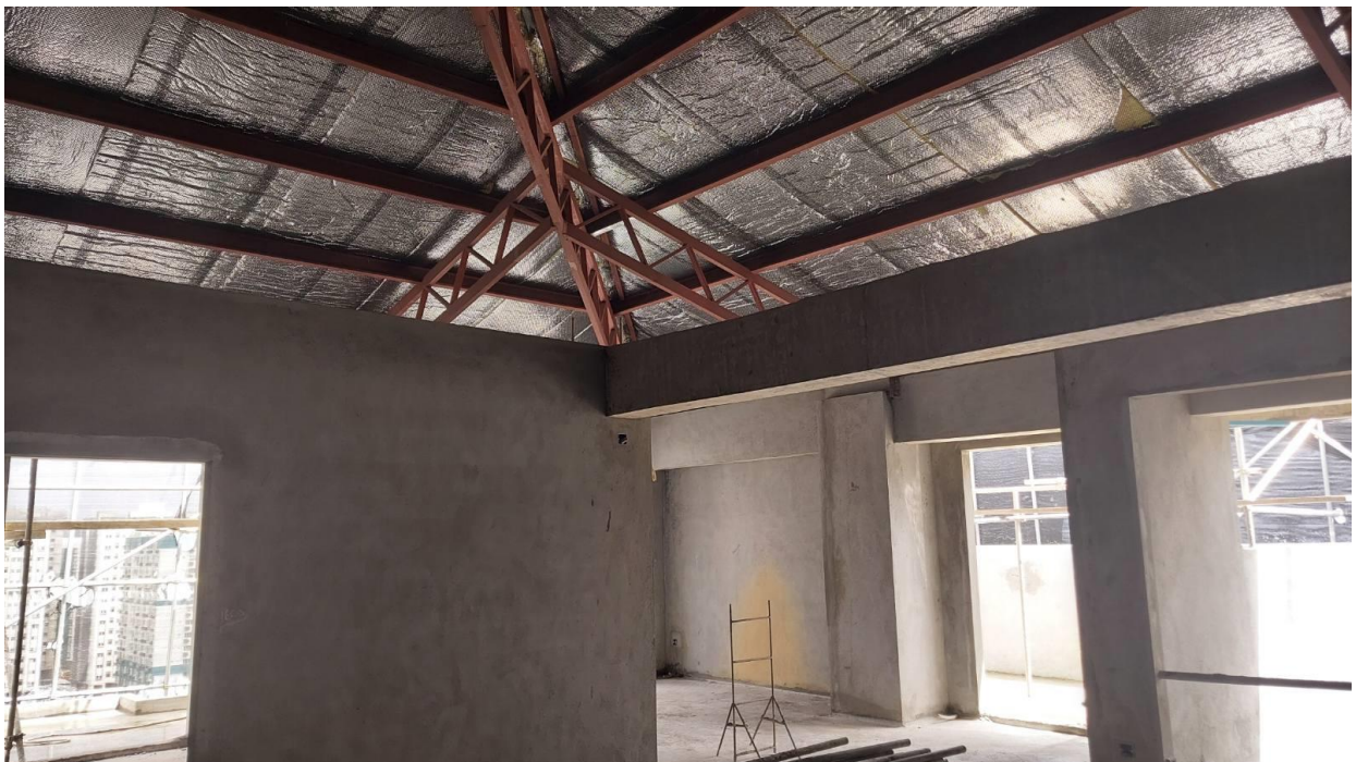
Penthouse internal plastering
