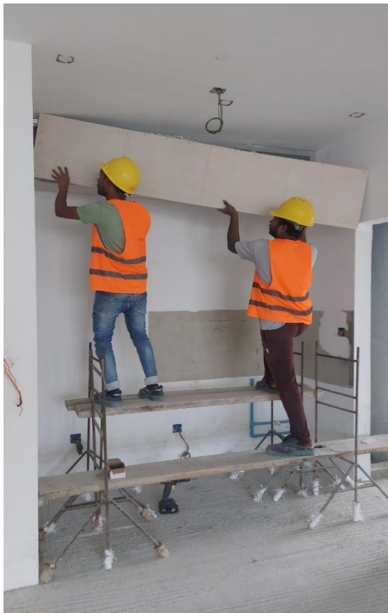
11 th floor Apartment ceiling board fixing
