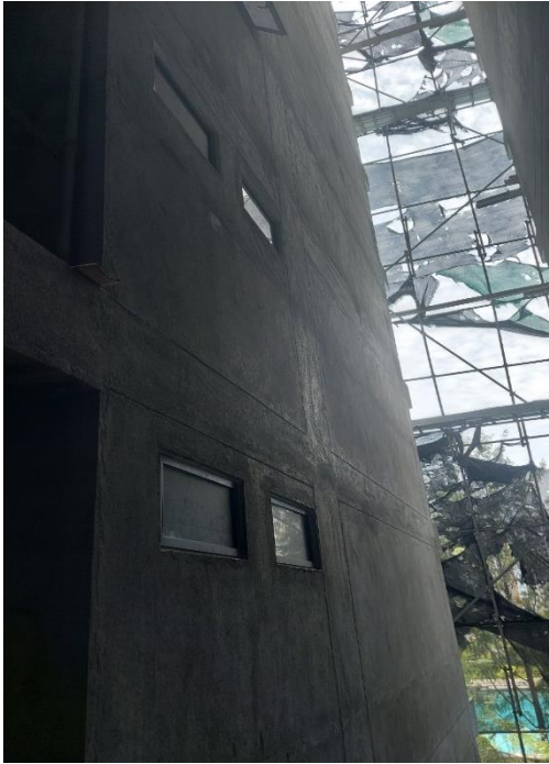
Front elevation air well area plastering
