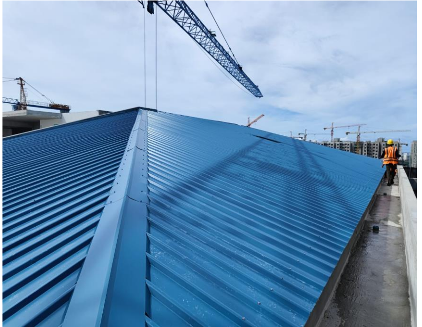
Roofing sheet laying
