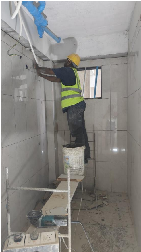
9 th floor tiling work
