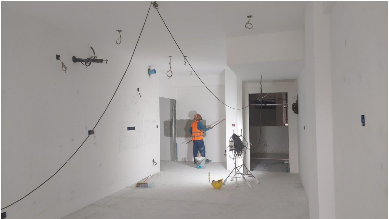
3 rd floor wiring, plumbing, ceiling and primer work
