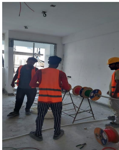
11 th floor wiring work
