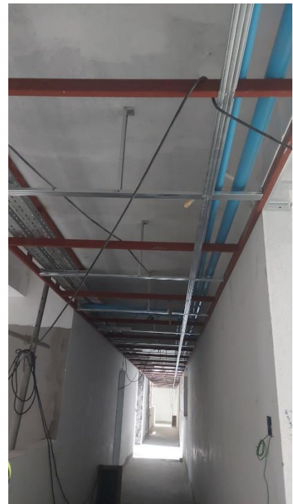
11 th floor common area ceiling work
