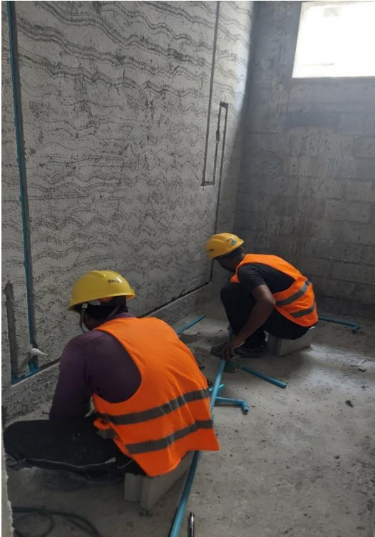
12 th floor plumbing work continuous
