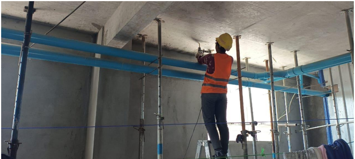
1 st floor plumbing work
