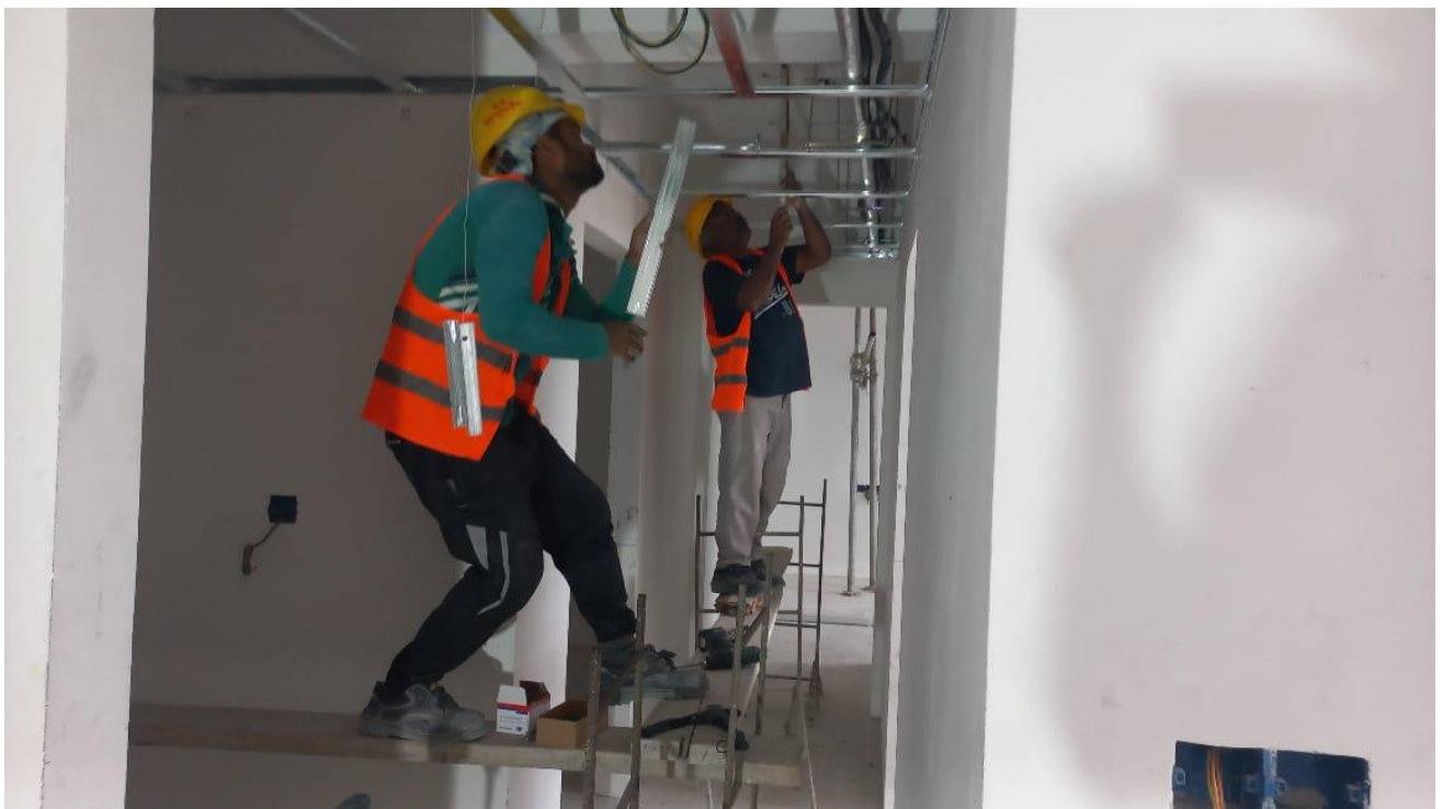
Common area and apartment false ceiling frame fixing
