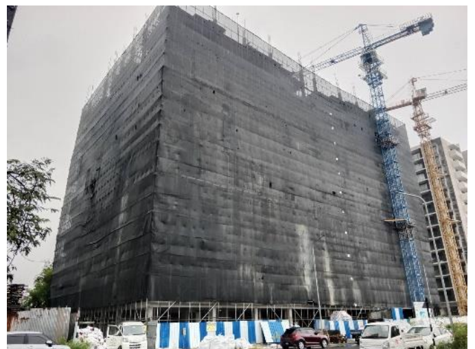
Safety Net Installation
