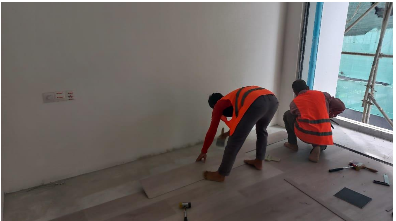
4 th floor SPC flooring laying
