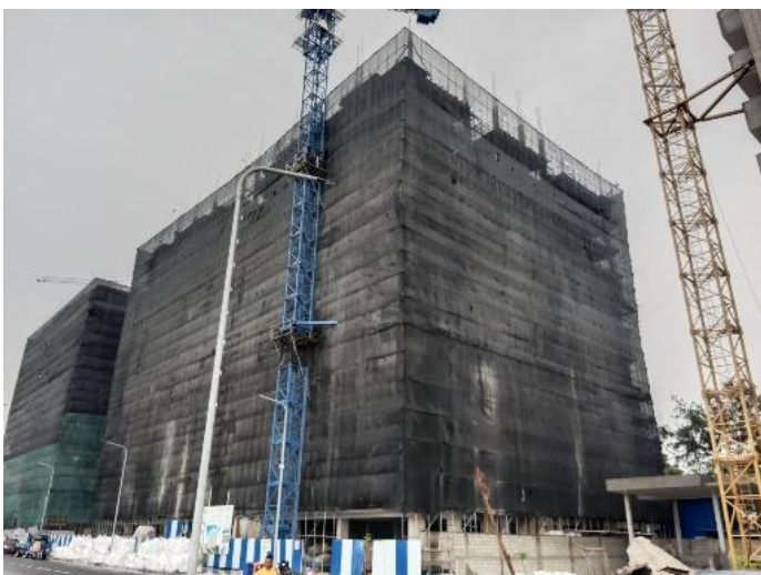
Safety Net installation
