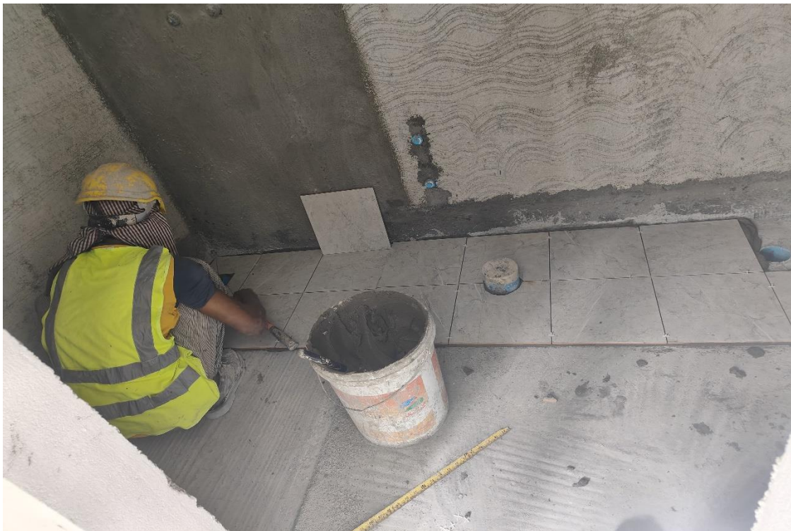
11 th floor toilet flooring tile work
