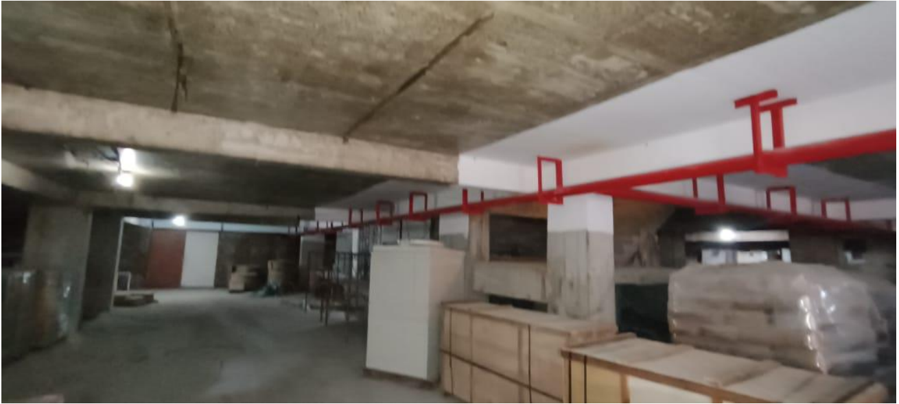
Fire line work
