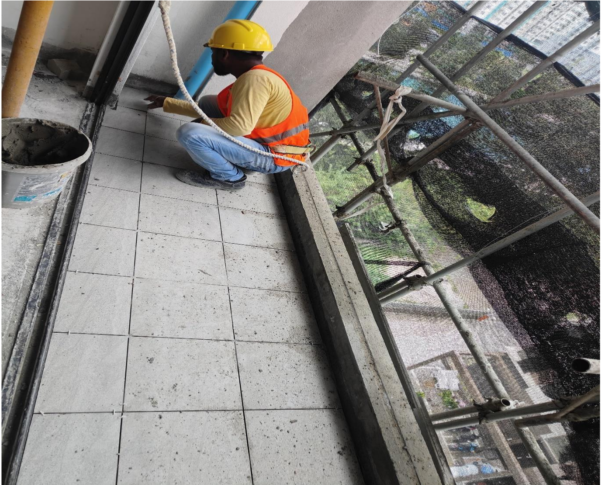
Balcony tile work
