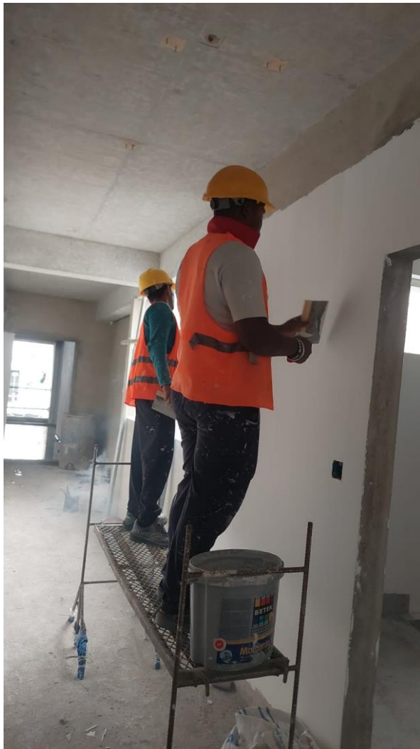
12 th floor putty work
