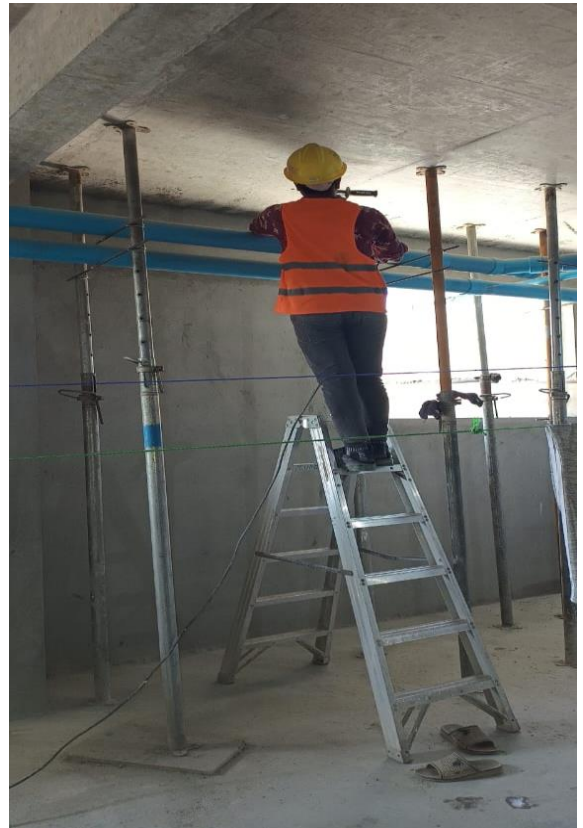
First floor plumbing work
