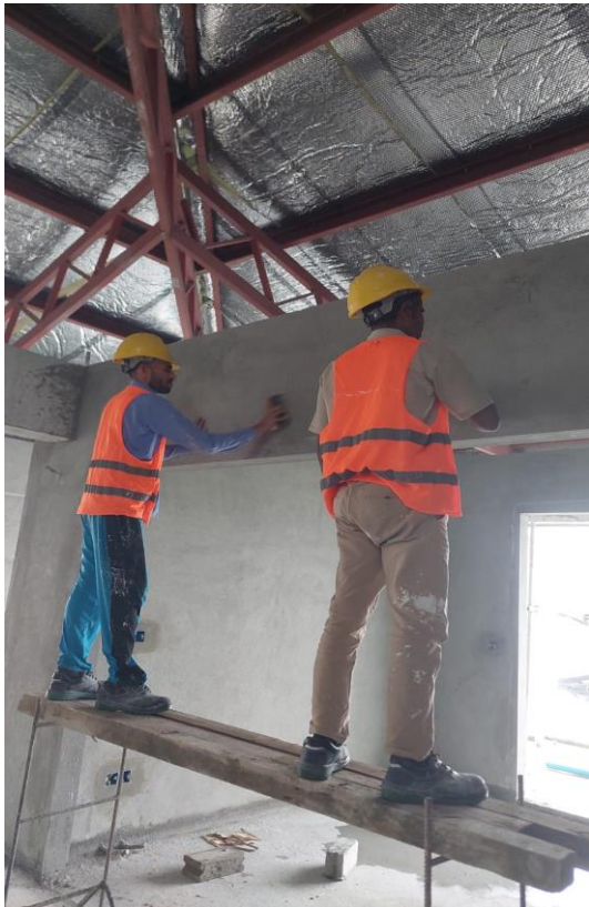
Penthouse putty work
