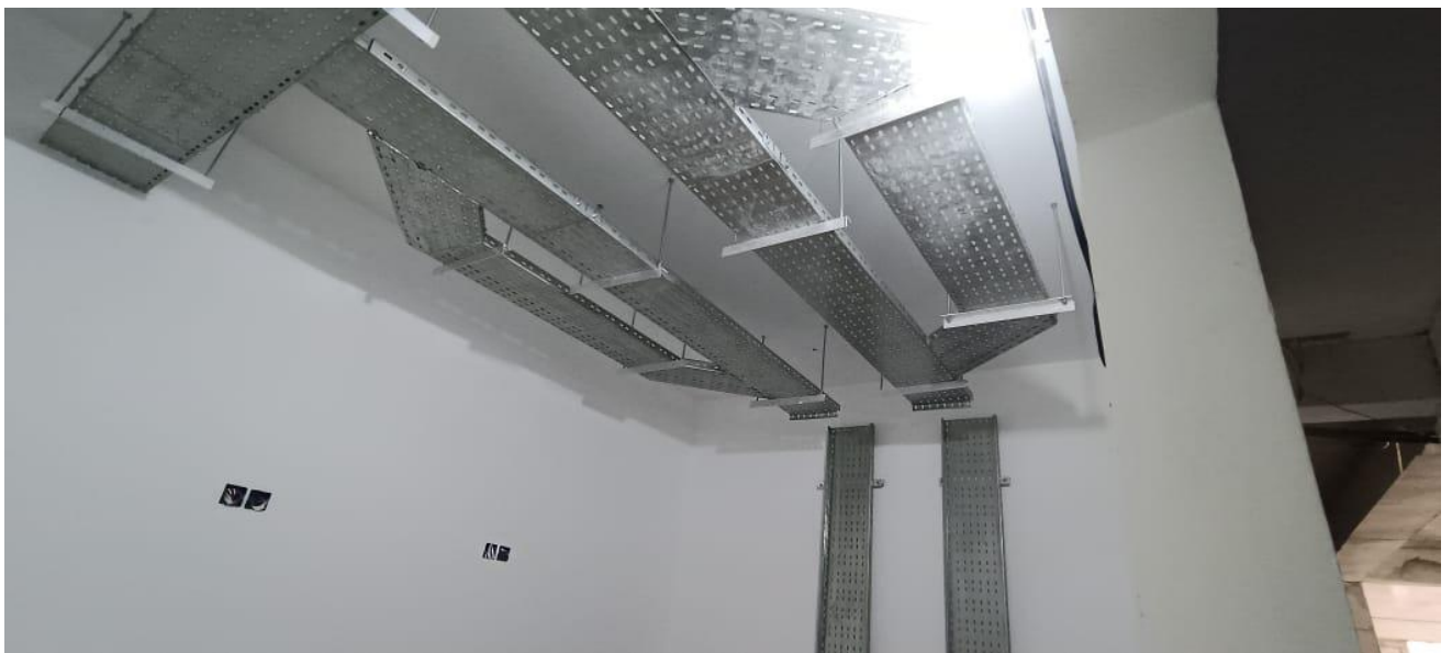
Cable tray fixing for cable laying
