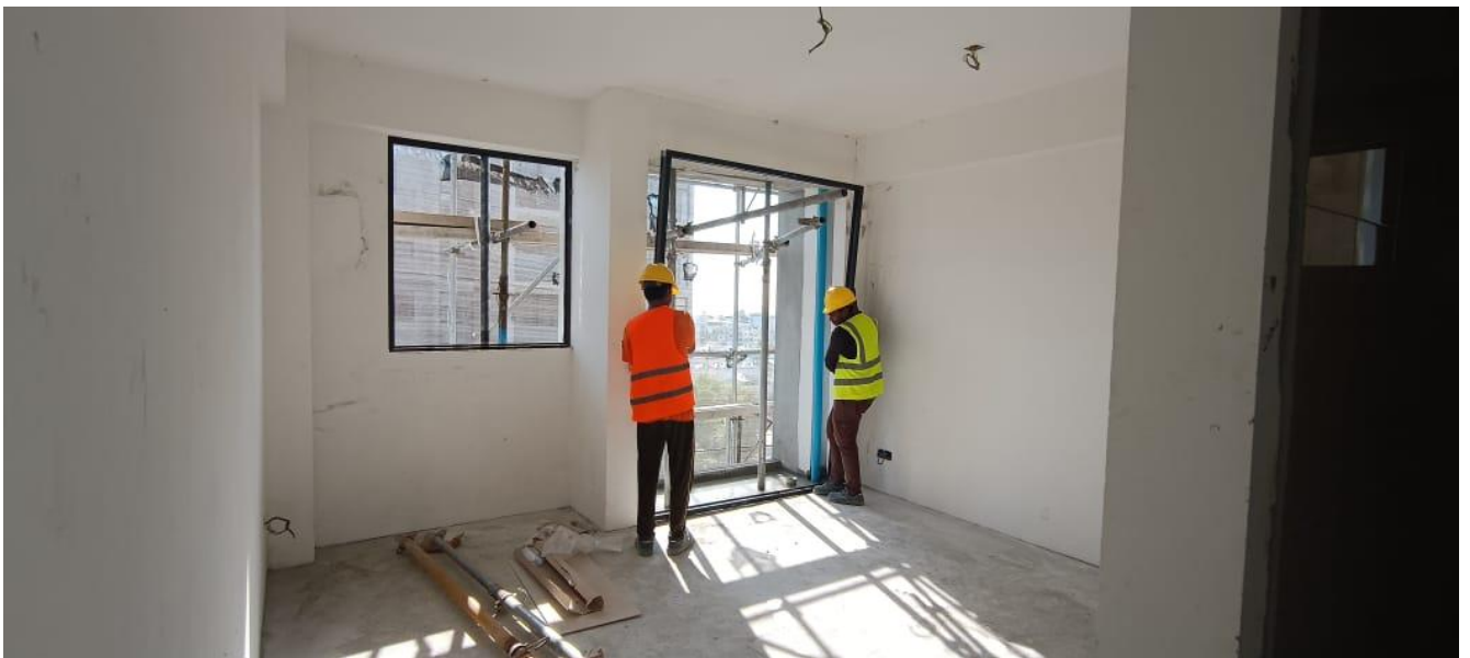
10 th floor sliding door fixing
