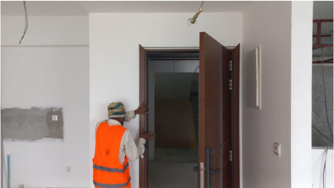
3 rd floor door fixing
