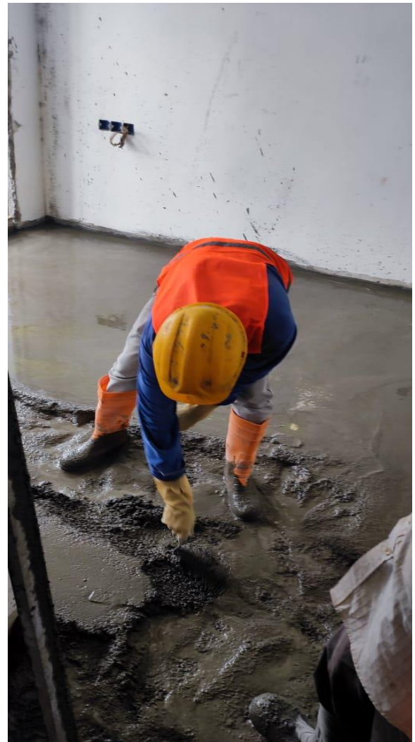
12 th floor screening work
