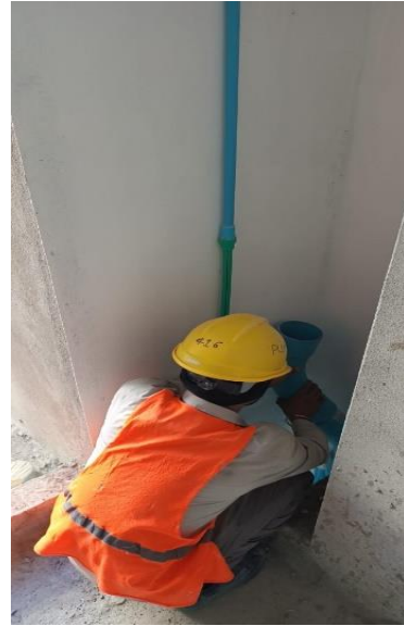
6 th floor plumbing work continues
