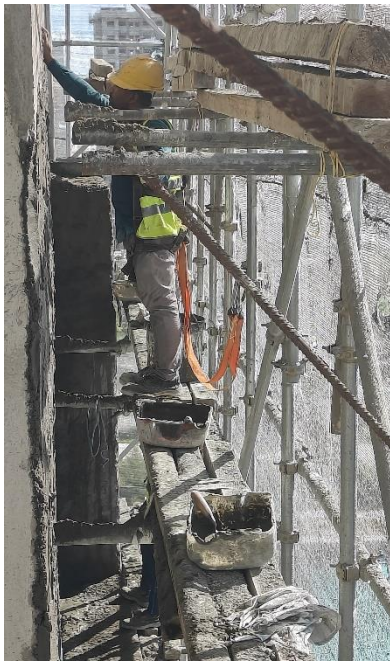
E apartment external plastering
