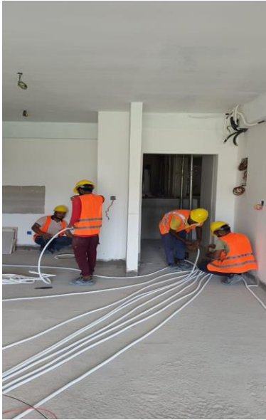
4 th floor floor wiring work continuous
