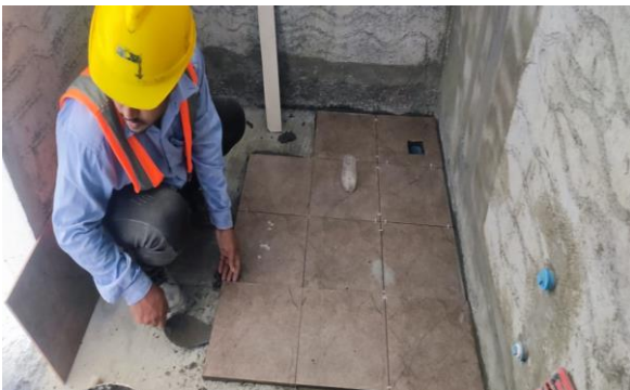
4 th floor toilet tile work
