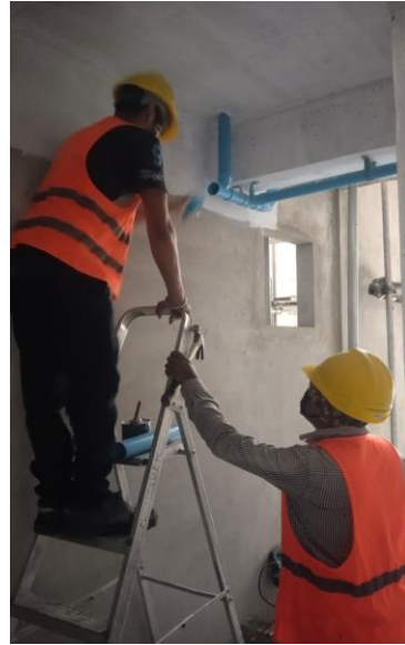
4 th floor plumbing work continues
