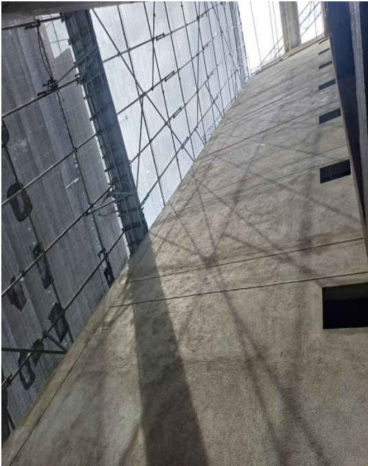
Elevation E5,E6 external plastering
