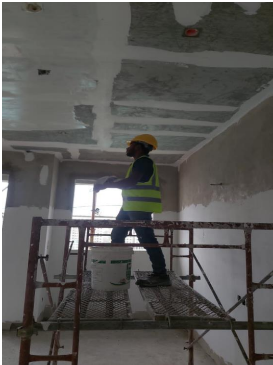
8 th floor wall and ceiling putty work
