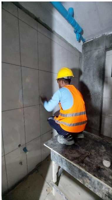
3 rd floor tile work
