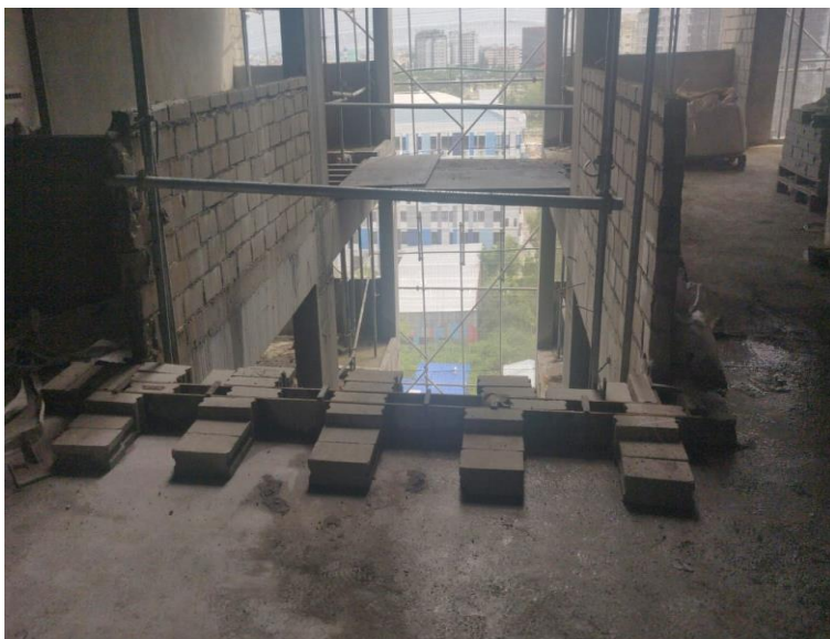
Common area wall kicker
