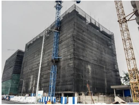
Safety Net installation
