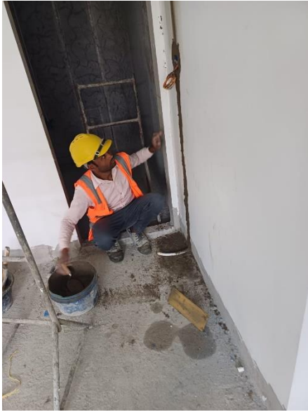
8 th floor socket box fixing
