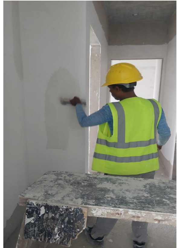
9 th floor wall and ceiling putty work
