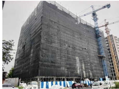
Safety Net Installation
