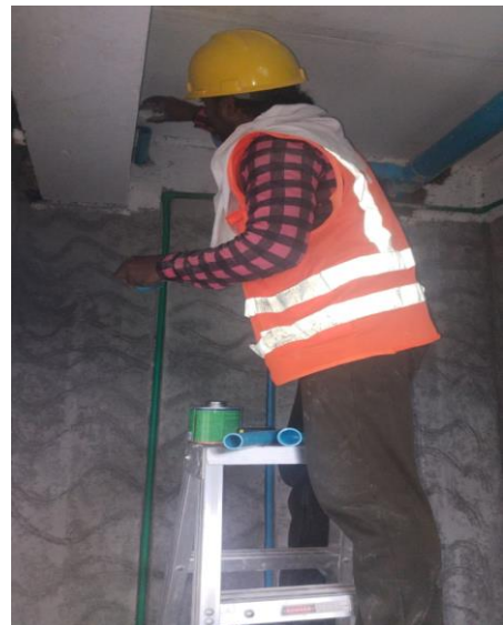
4 th floor toilet plumbing work
