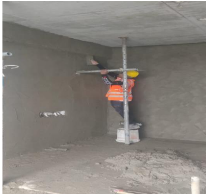
7 th floor plastering
