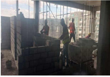
10 th floor block works
