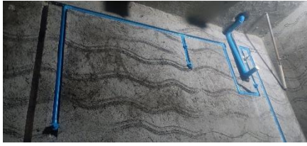
5 th floor plumbing work
