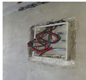
5 th floor type C wiring work
