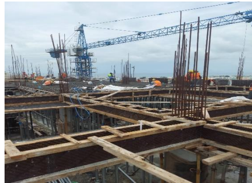
Roof terrace beam form work
