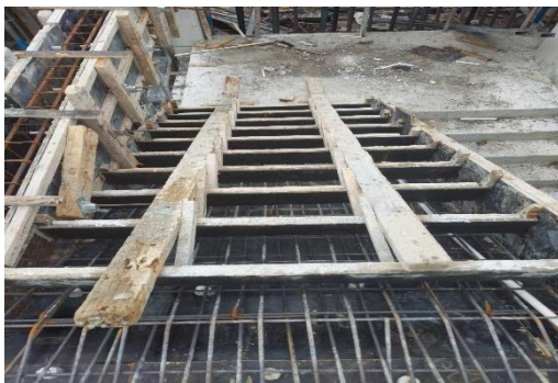
13 to roof terrace stair reinforcement
