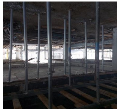
12th Floor de shuttering
