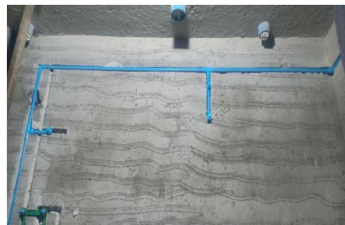
5 th floor type B plumbing work
