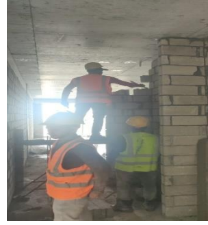
10th Floor Blocks Laying
