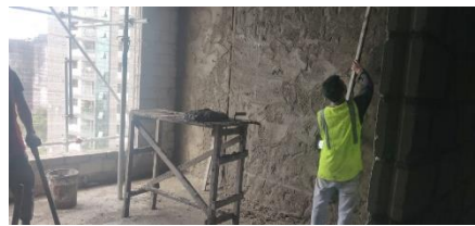
8 th floor plastering
