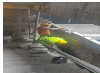
9 th floor block work
