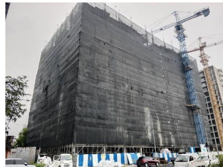
Safety Net Installation
