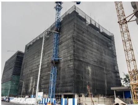
Safety Net installation
