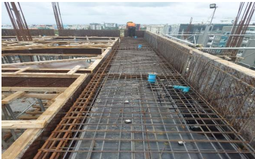
Roof terrace Electrical & Plumbing Sleeve
