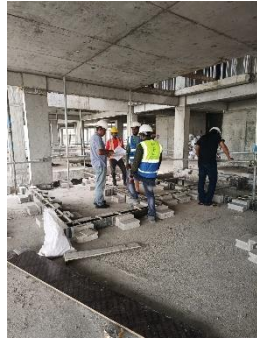
10 th floor kicker inspection
