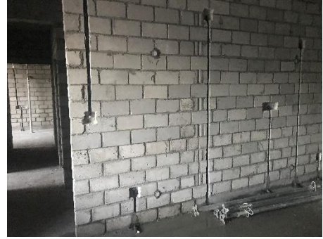
5th Floor Blocks Laying
