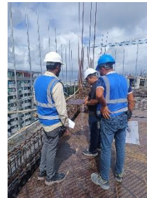
13th Floor Beam Reinforcement
