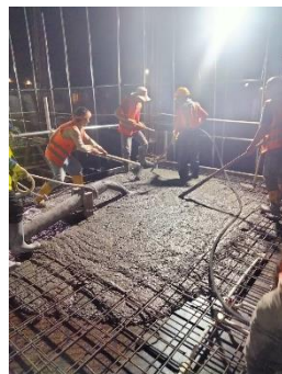
13th Floor Slab casting work
