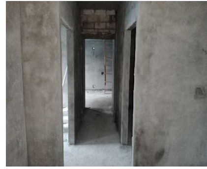
6 th floor Plastering
