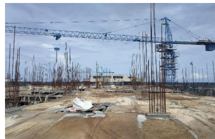
13th Floor Slab Concrete Curing
