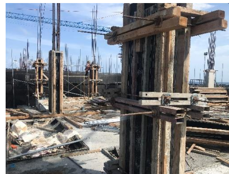
13th Floor Column Formworks
