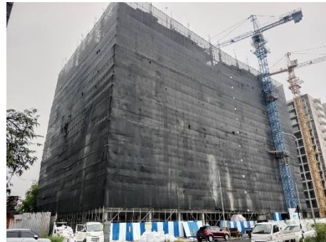
Safety Net Installation
