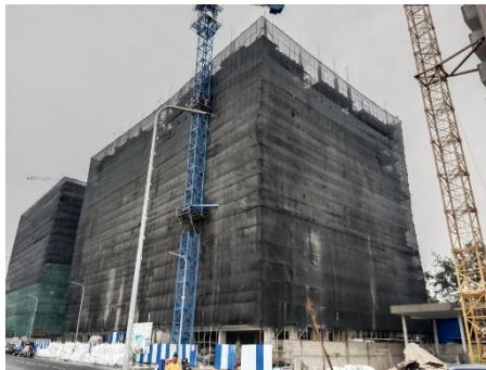
Safety Net installation
