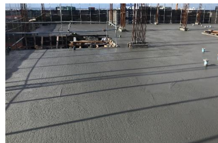
13th Floor slab casting
