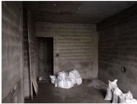
6 th floor plastering
