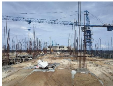
13th Floor Slab Casted.
