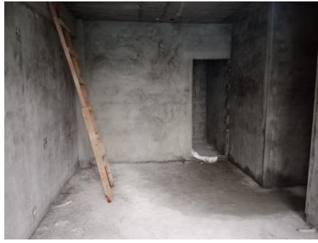
5 th floor Plastering
