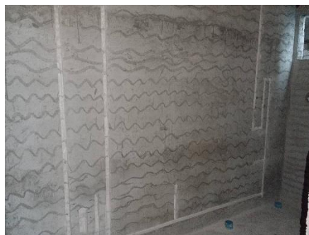
5 th floor plumbing wall chasing
