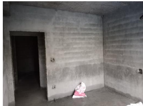
7 th floor plastering
