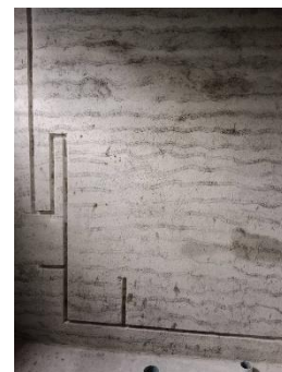
6 th floor plumbing wall chasing
