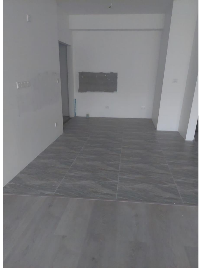
3 rd floor kitchen floor tile laying
