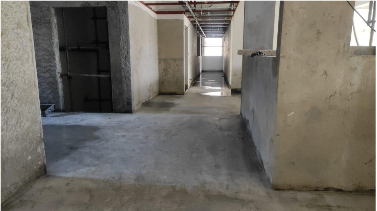
3 rd floor common area screeding
