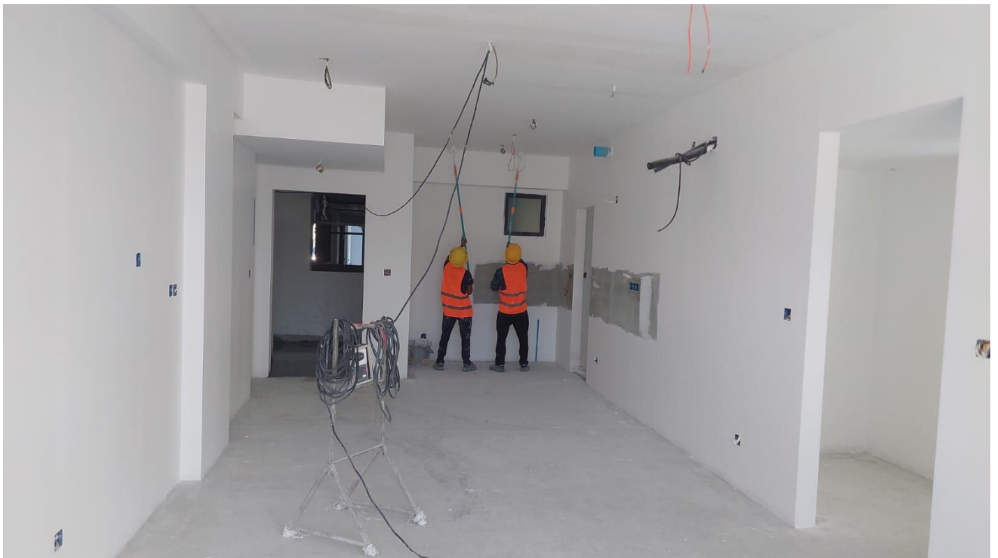
3 rd floor primer and emulsion painting work
