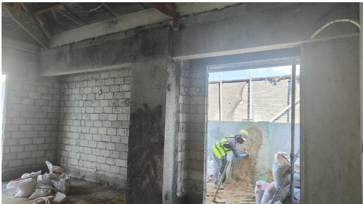
13 th floor block work
