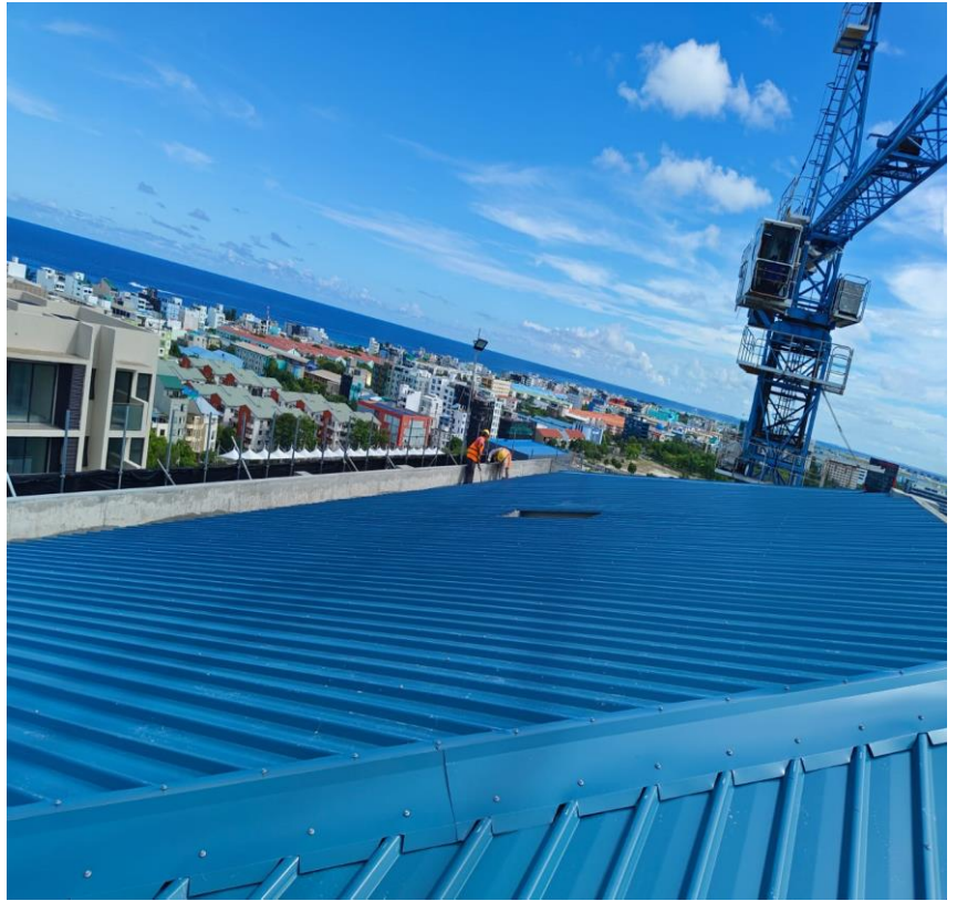
Roofing sheet laying
