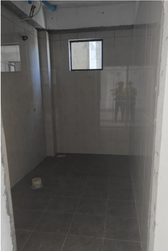
11 th floor tiling work
