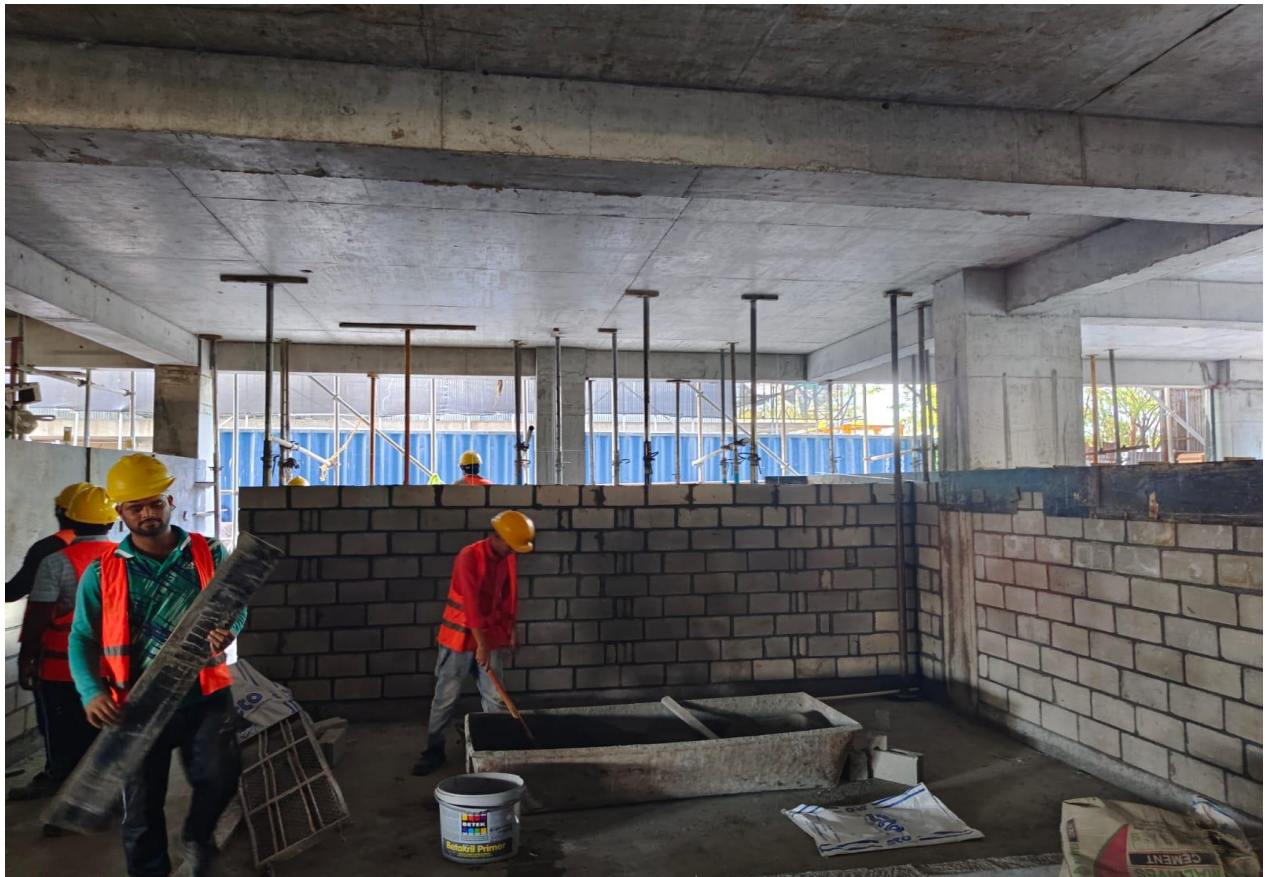
Ground floor electrical room block work
