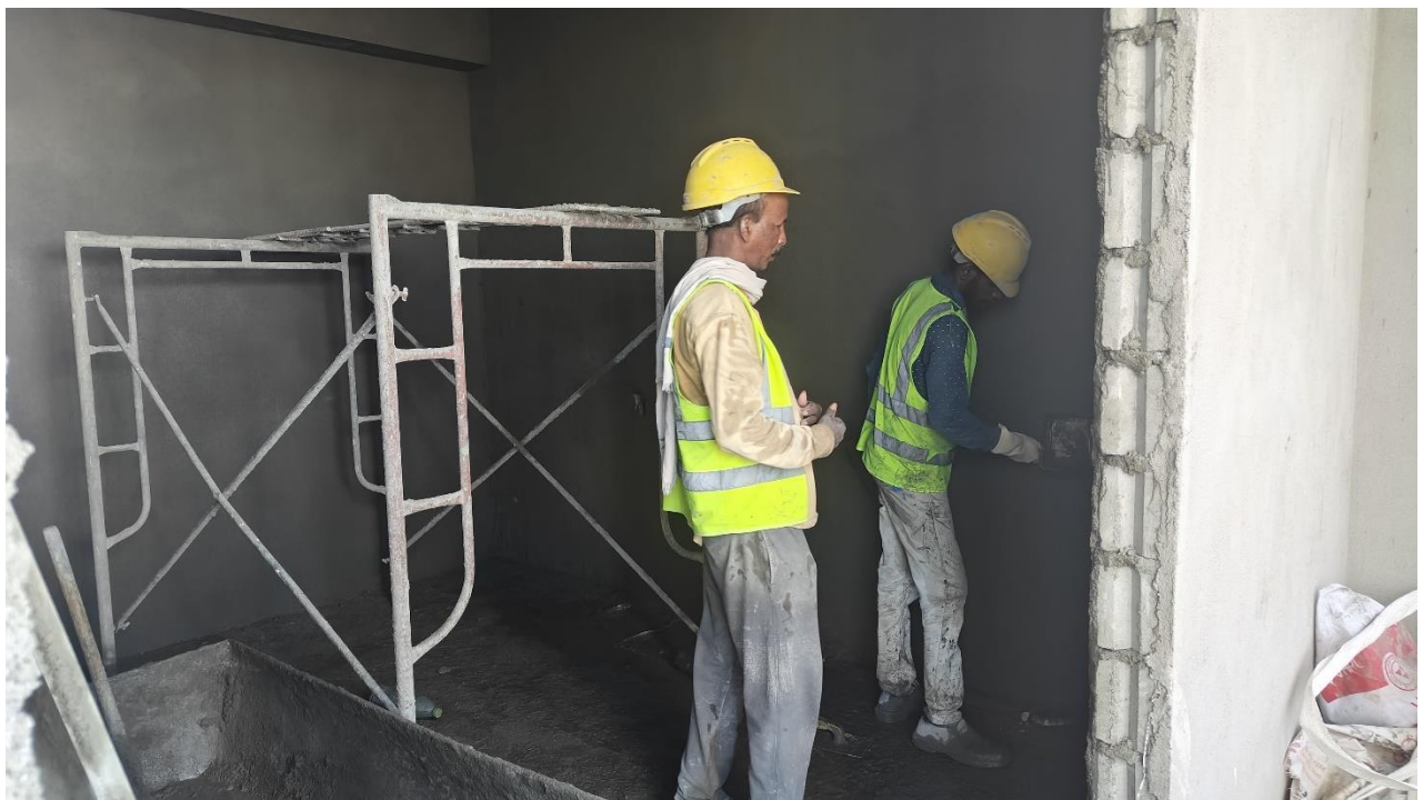
13 th floor internal plastering
