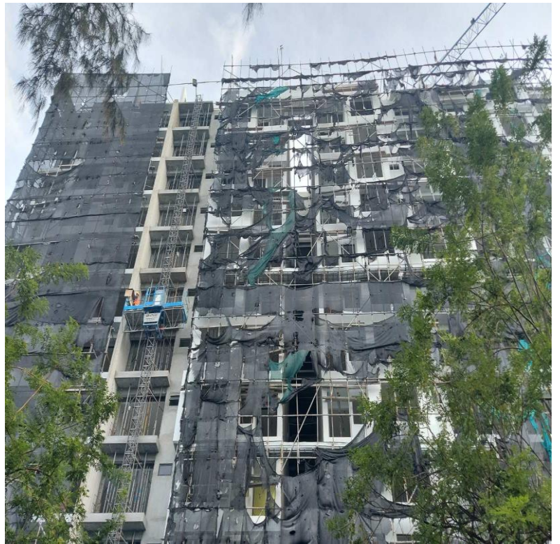
2 nd to 13 th floor ex painting work
