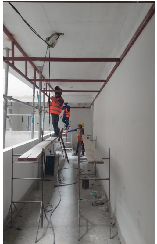
7 th floor common area ceiling work
