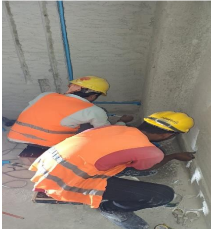
11 th floor plumbing work continuous
