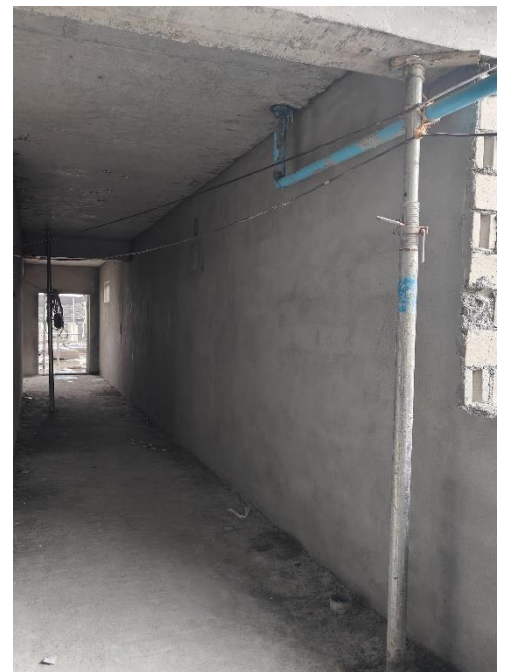
Terrace floor common area plastering
