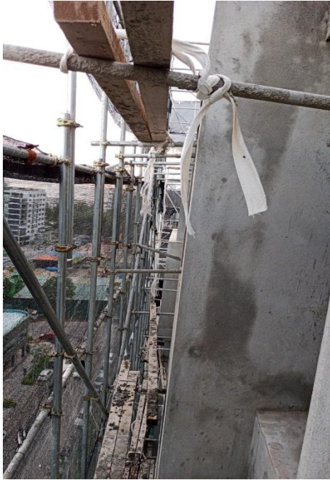
E 2 external wall plastering
