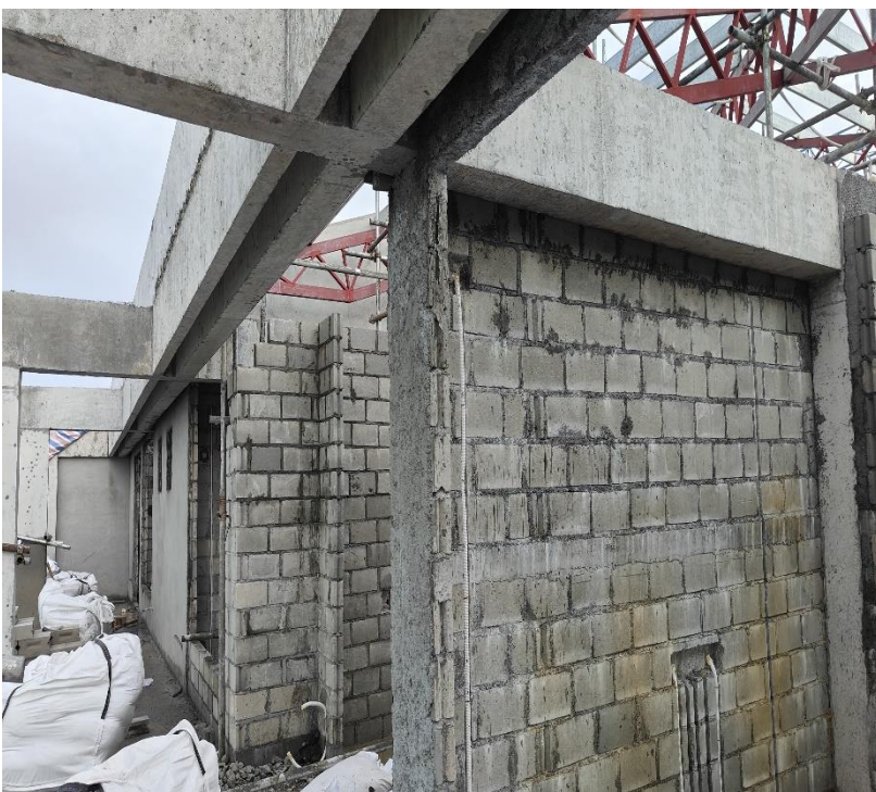
13 th floor block work
