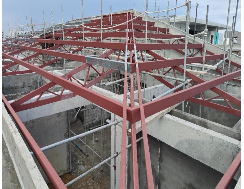
Roof purlin erection and primer
