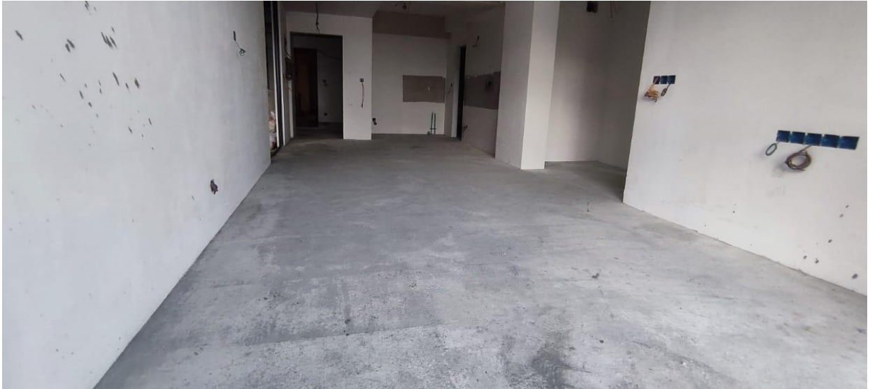
6 th floor screeding work
