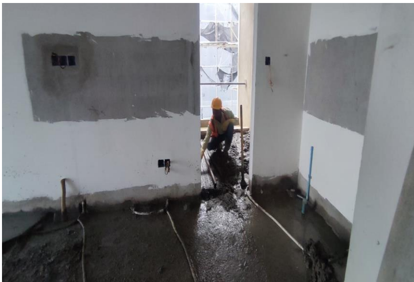
6 th floor screeding work
