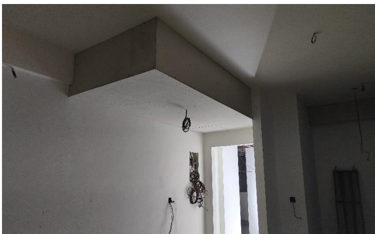
6 th floor ceiling work
