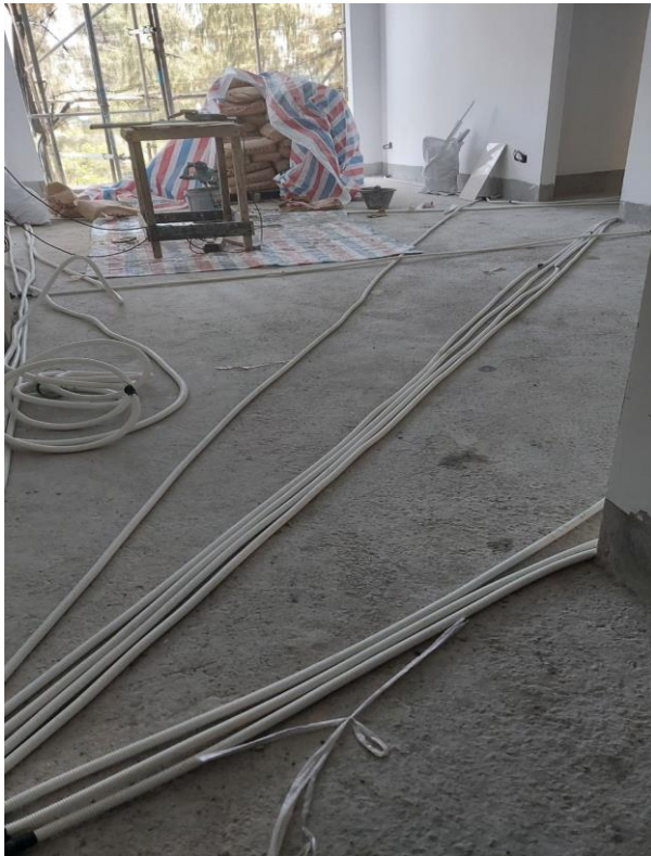
9 th floor floor wiring
