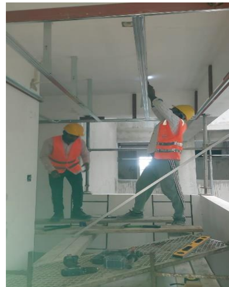
8 th floor ceiling work
