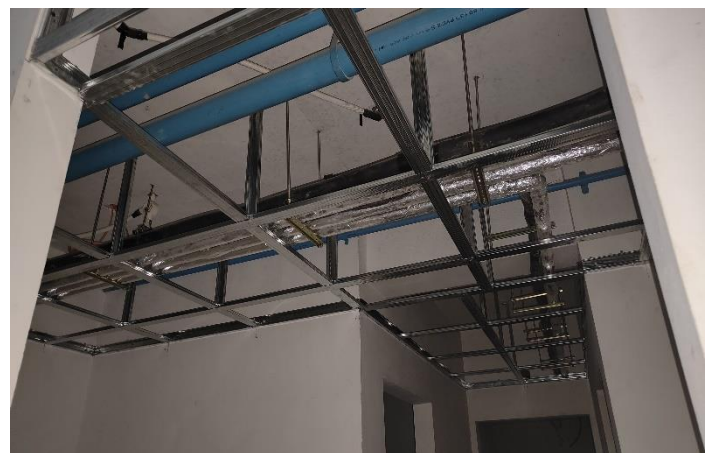
7 th floor Ac and plumbing work
