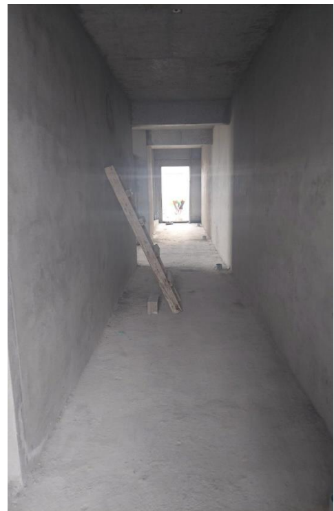
Terrace floor common area plastering
