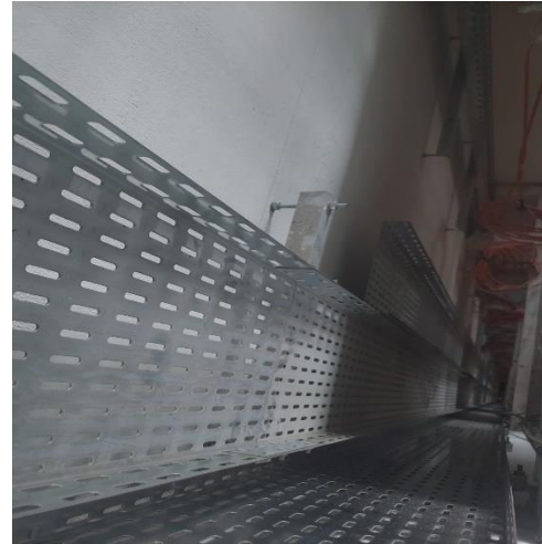
2 nd to 12 th floor cable tray laying
