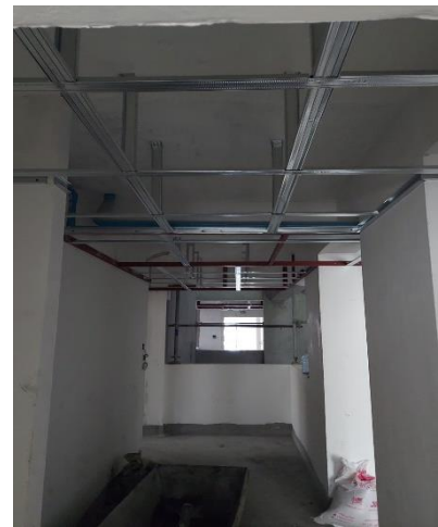
7 th floor ceiling work
