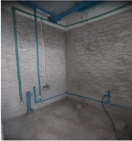
10 th floor plumbing work continuous
