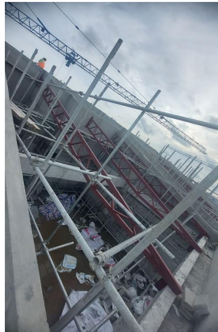
Roof truss erection
