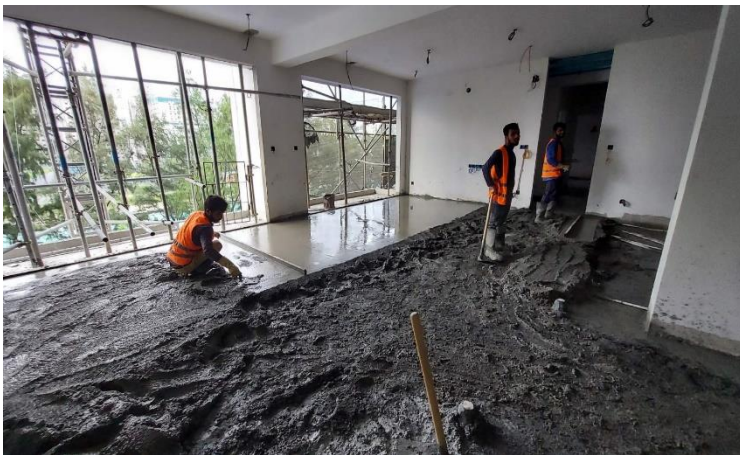
4 th floor screeding work
