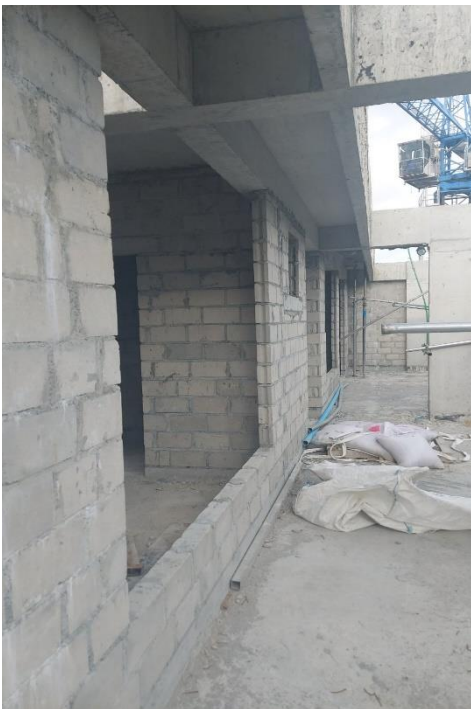
13 th floor block work
