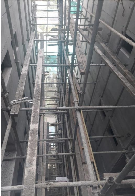
C D air well external wall plastering
