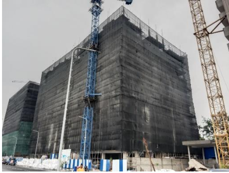
Safety Net installation
