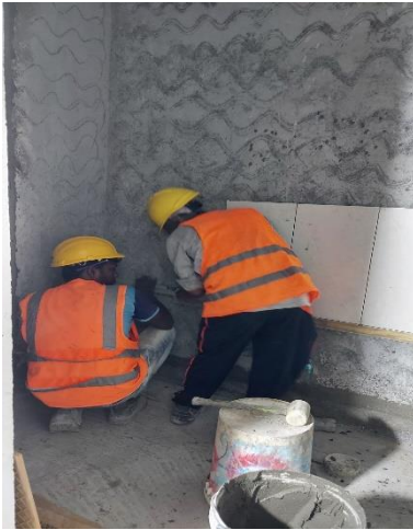
6 th floor toilet tile work
