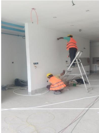
6 th floor floor wiring work continuous
