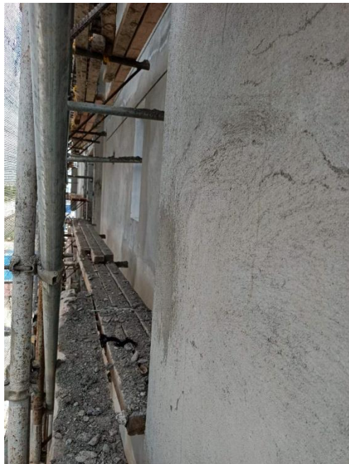
J apartment external plastering
