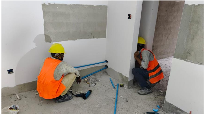
7 th floor plumbing work continues
