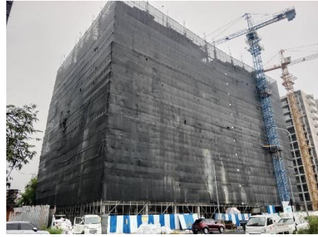
Safety Net Installation
