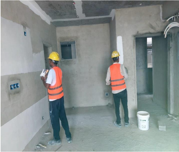
10 th floor wall and ceiling putty work
