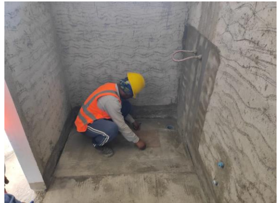
5 th floor toilet tile work
