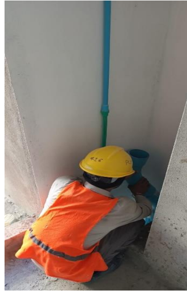
6 th floor plumbing work continues
