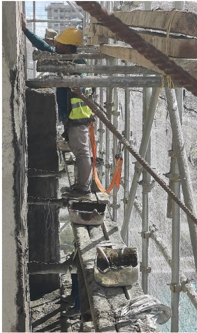
E apartment external plastering
