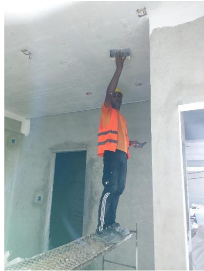
11 th floor wall and ceiling putty work
