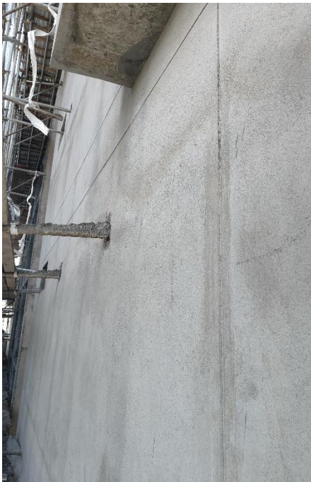
G apartment external plastering
