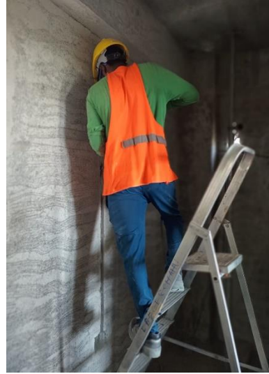
6 th floor plumbing work continues
