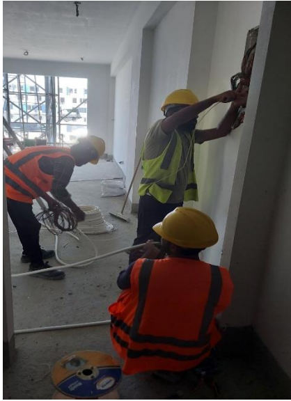
3 rd floor floor wiring work continuous
