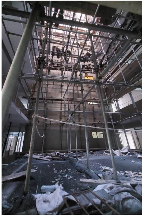
D and G air well external plastering
