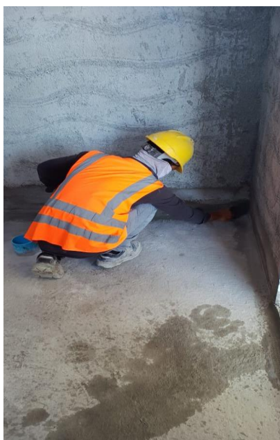
4 th floor water proofing work
