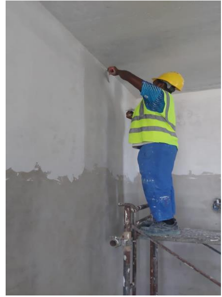
10 th floor wall and ceiling putty work
