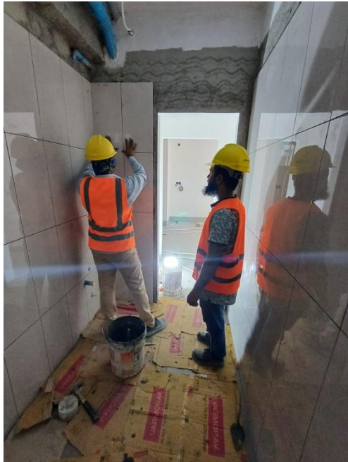
3 rd floor B toilet wall and floor tile work
