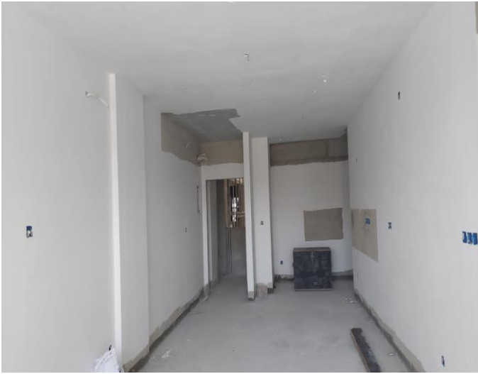
8 th floor wall and ceiling putty work
