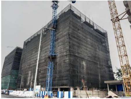
Safety Net installation
