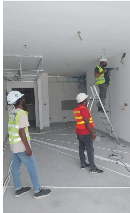
3 rd floor AC installation work
