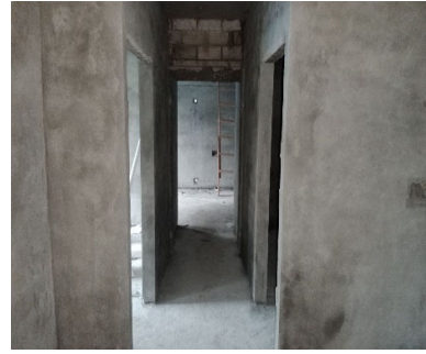
6 th floor Plastering
