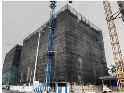
Safety Net installation
