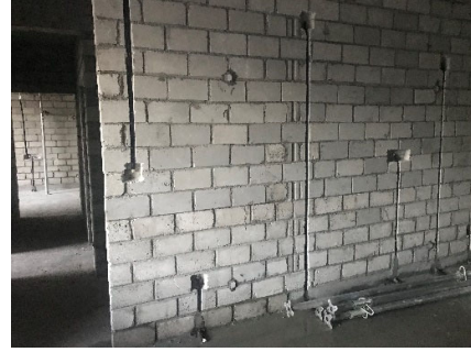
5th Floor Blocks Laying
