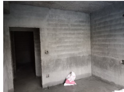
7 th floor plastering
