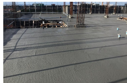
13th Floor slab casting
