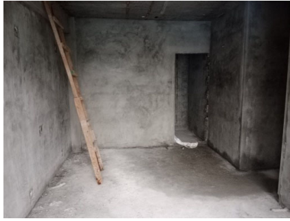
5 th floor Plastering
