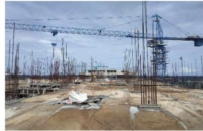
13th Floor Slab Concrete Curing
