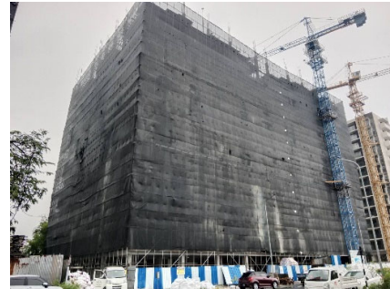
Safety Net Installation
