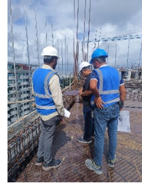
13th Floor Beam Reinforcement
