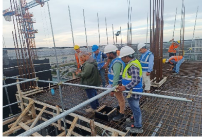
13th Floor Slab Reinf.
