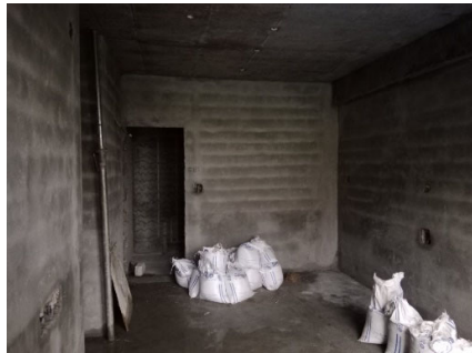
6 th floor plastering
