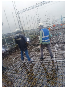
13th Floor Electrical & Plumbing Sleeve
