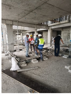
10 th floor kicker inspection
