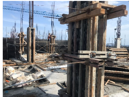
13th Floor Column Formworks
