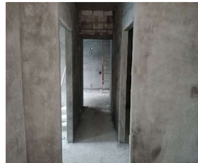
3 rd floor Plastering
