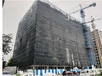
Safety Net Installation
