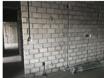
4th Floor Blocks Laying
