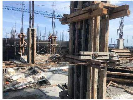
12th Floor Column Formworks
