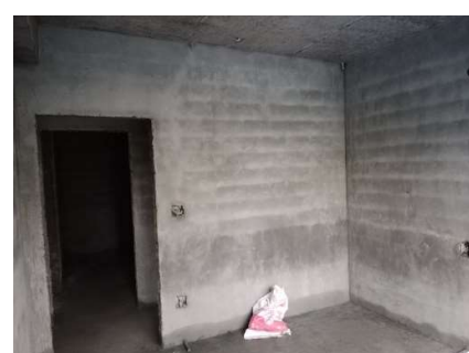
3rd floor plastering
