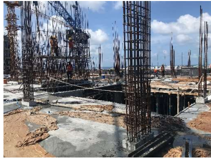
12th Floor Column Reinforcement
