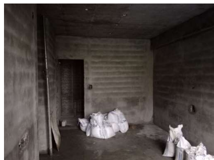
3rd floor plastering
