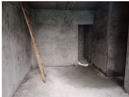
2 nd floor Plastering
