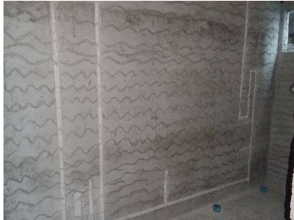
3 rd floor plumbing wall chasing
