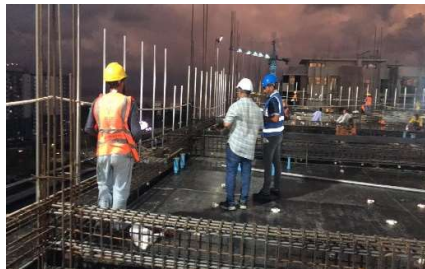
12th Floor Beam & Slab Reinf.
