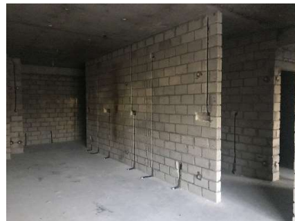
3rd Floor Electrical Wall Chasing
