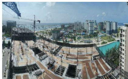
10th Floor Slab Concrete Casting
