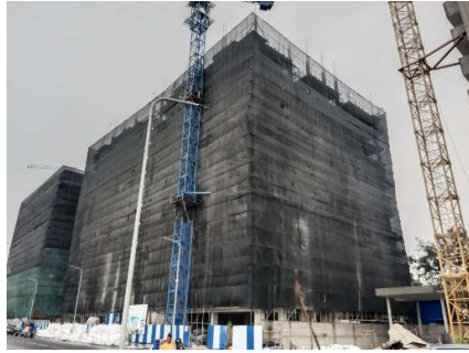
Safety Net installation
