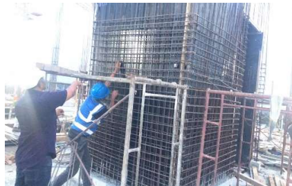
12th Floor Lift wall Reinforcement
