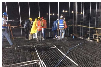
10th Floor Electrical & Plumbing Sleeve
