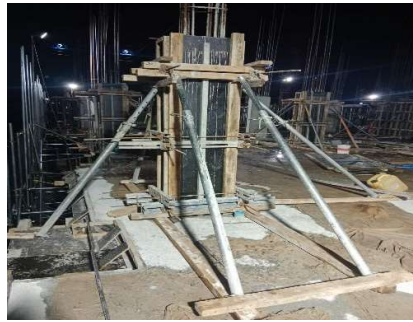
12th Floor Columns Concrete Casting
