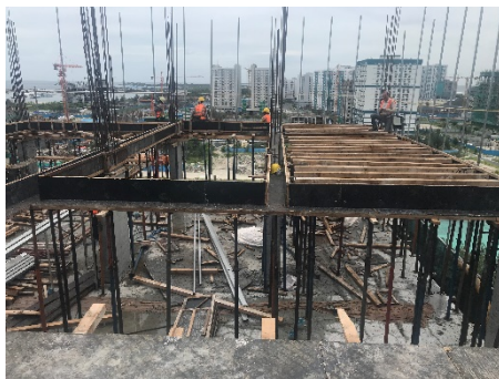
10th Floor Beam & Slab Reinf.
