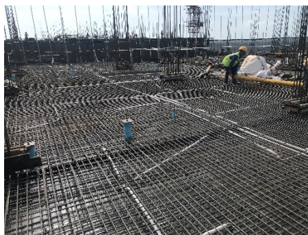
11th Floor Slab Reinforcement
