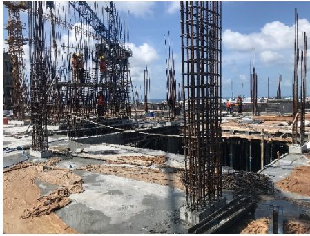
10th Floor Column Reinforcement
