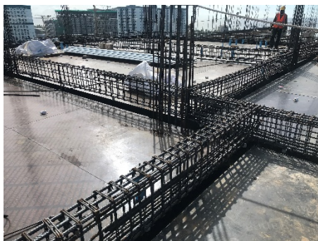
11th Floor Beam Reinforcement
