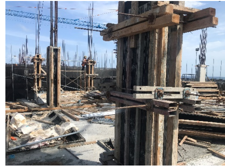
10th Floor Column Formworks
