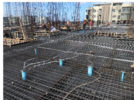
11th Electrical & Plumbing Sleeve
