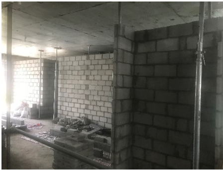
5th Floor Blocks Laying
