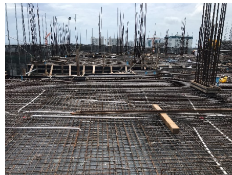
10th Floor Beam & Slab Formworks
