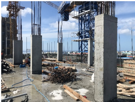
10th Floor Columns Concrete Casting
