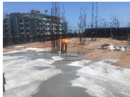
10th Floor Slab Concrete Casting
