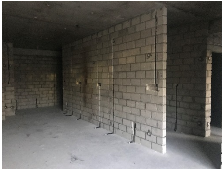
3rd Floor Electrical Wall Chasing
