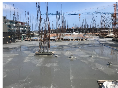
11th Floor Slab Concrete Casting
