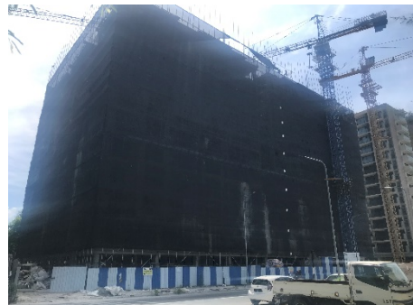
Safety Net Installation
