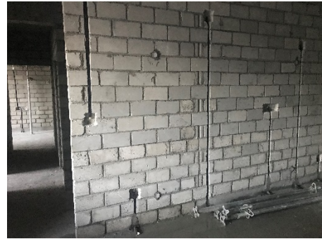
4th Floor Blocks Laying
