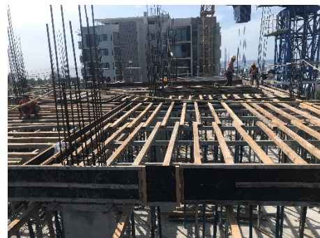
11th Floor Beam & Slab Formworks
