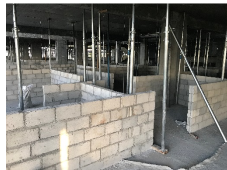
4th Floor Blocks Laying
