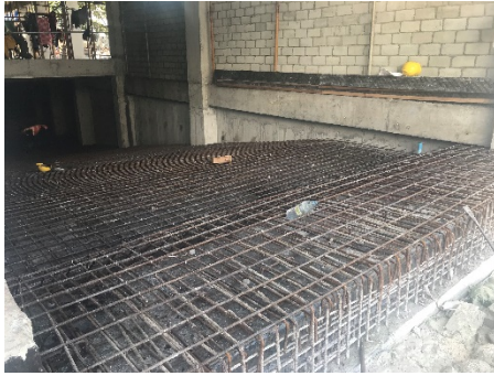
Basement Ramp Reinforcement
