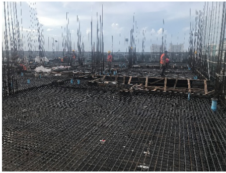
8th Floor Beam & Slab Reinforcement
