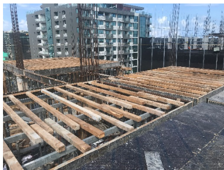
9th Floor Beam & Slab Formworks
