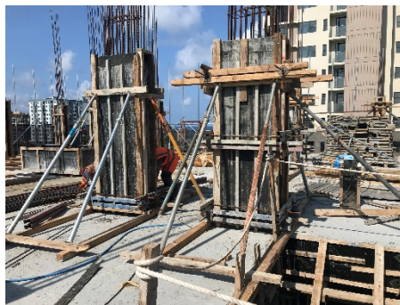
8th Floor Column Formworks
