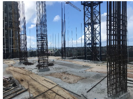
8th Floor Column Reinforcement
