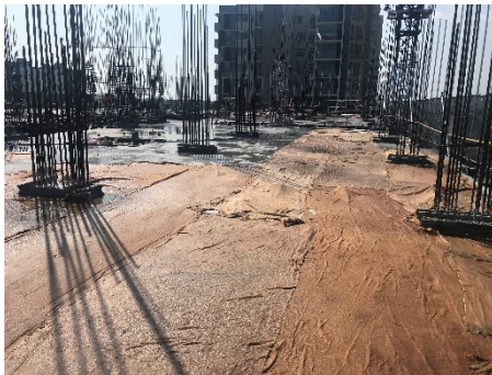
8th Floor Slab Concrete Casting
