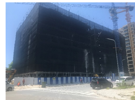
Safety Net Installation
