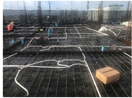
8th Floor Plumbing & Electrical Sleeve
