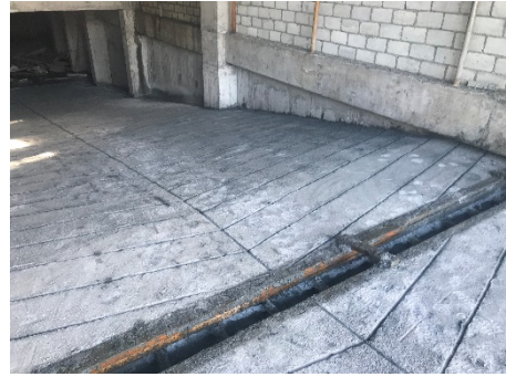
Basement Ramp Concrete Casting
