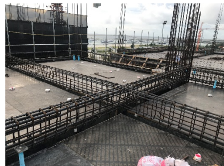
9th Floor Beam Reinforcement
