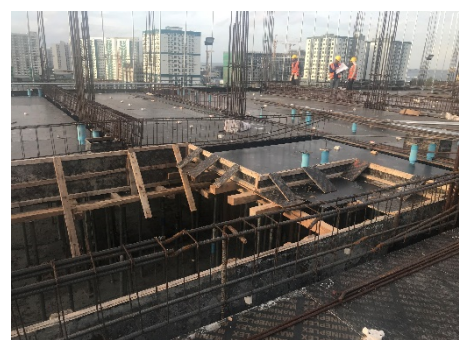
8th Floor Beam Reinforcement
