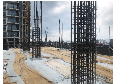
7th Floor Column Reinforcement
