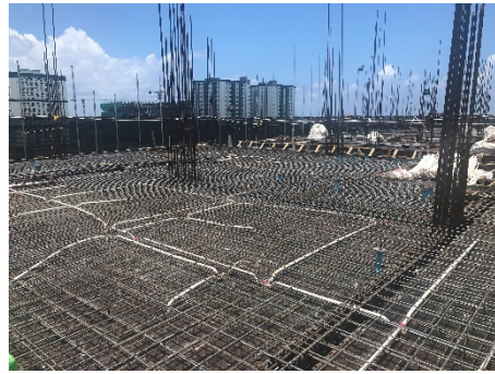
7th Floor Beam & Slab Reinforcement
