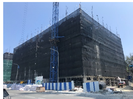
Safety Net Installation
