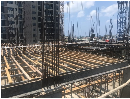
7th Floor Beam & Slab Formworks
