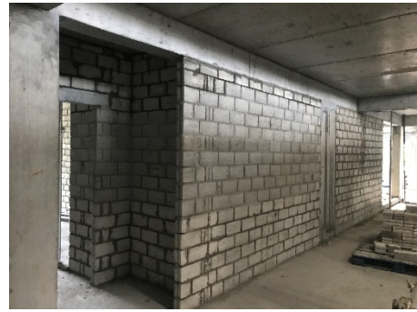
2nd Floor Blocks Laying
