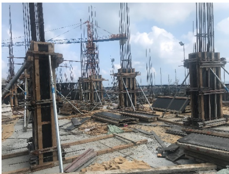
7th Floor Column Formworks
