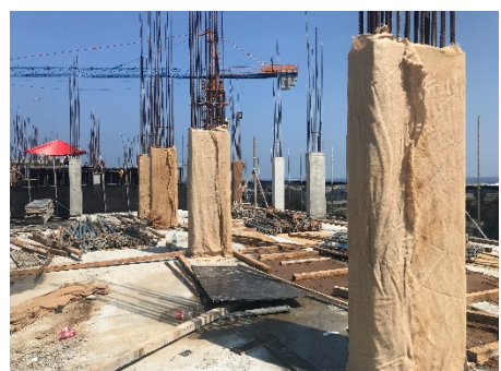
7th Floor Column Concrete Casting
