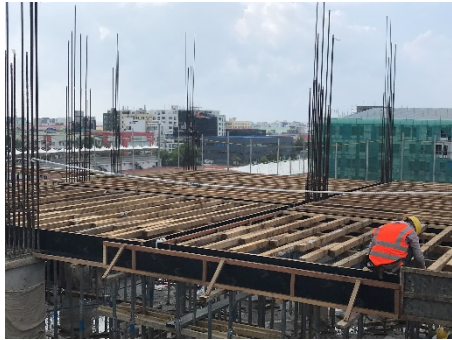
6th Floor Beam & Slab Formworks
