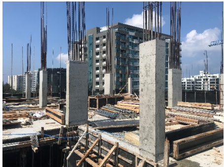
6th Floor Column Concrete Casting
