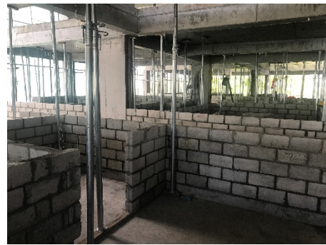
2 nd Floor Block Laying
