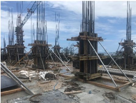
6th Floor Column Formworks
