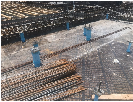
7 th Floor Plumbing Sleeve Installation
