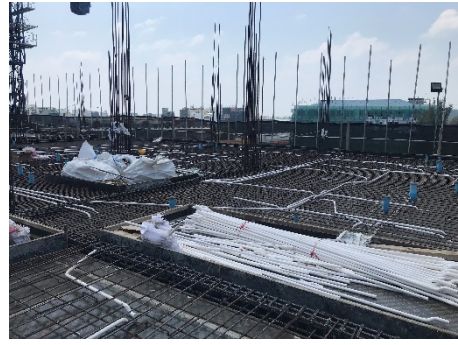
7 th Floor Electrical Sleeve Installation
