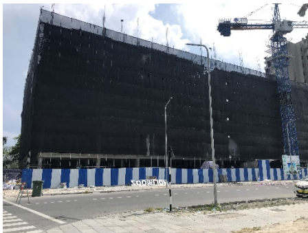
Safety Net Installation
