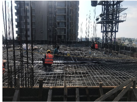
6th Floor Beam & Slab Reinforcement
