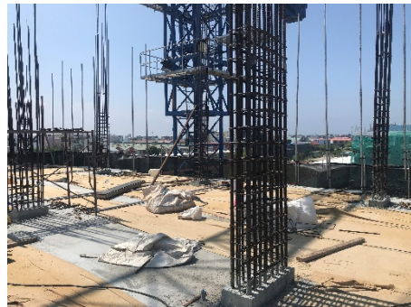
6th Floor Column Reinforcement
