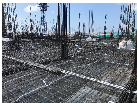
7th Floor Beam & Slab Reinforcement
