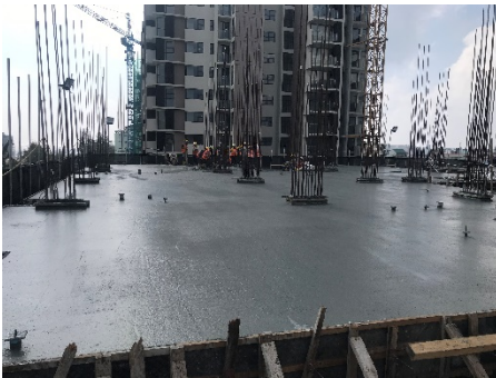
6th Floor Slab Concrete Casting
