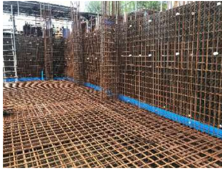
Water Bar Installation
