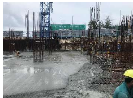
Foundation Raft and Beam Casting
