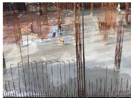
Foundation Raft and Beam Casting
