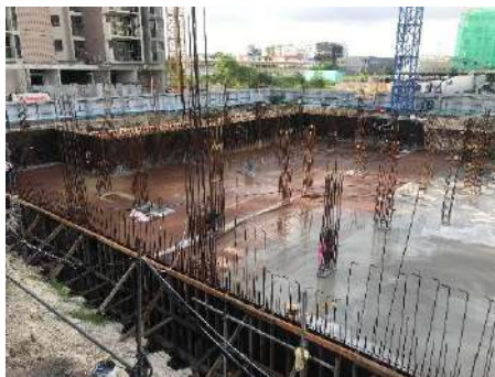
Foundation Raft and Beam Casting
