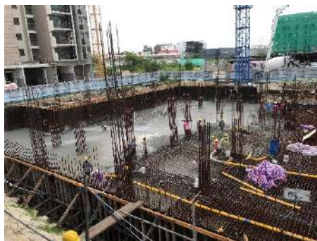
Foundation Raft and Beam Casting
