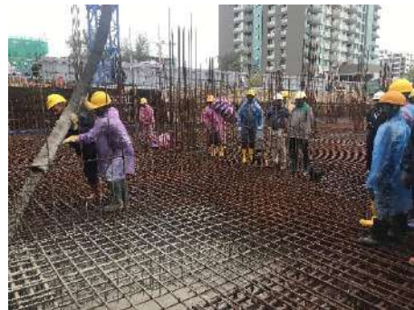
Foundation Raft and Beam Casting
