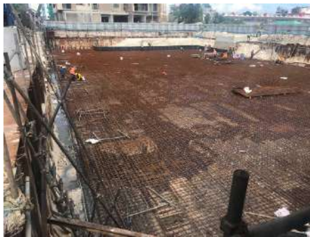
Raft Reinforcement
