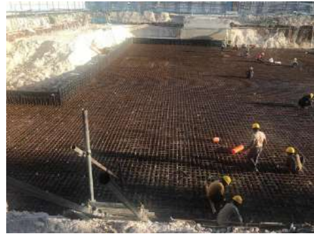
Raft Reinforcement
