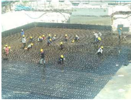
Raft Reinforcement
